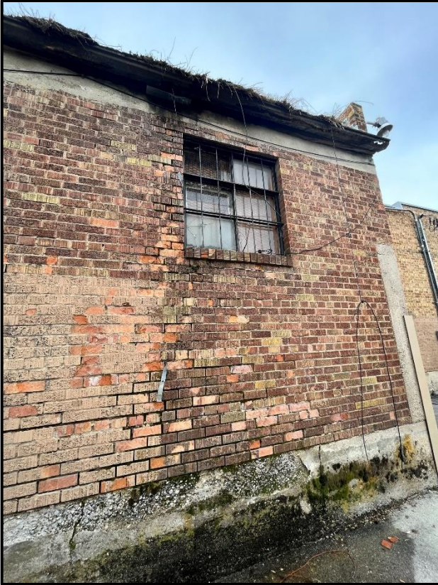
Rear wall to be demolished
