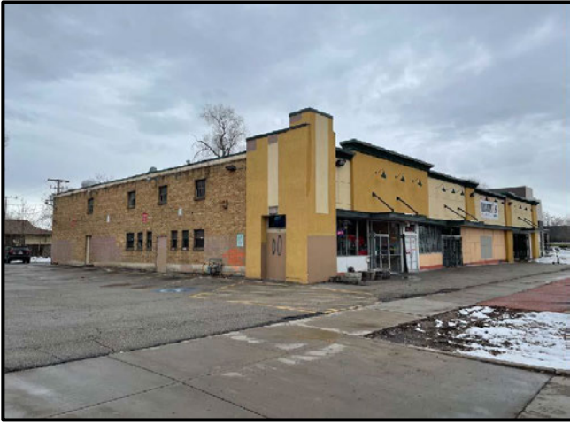
Subject site, facing southwest
