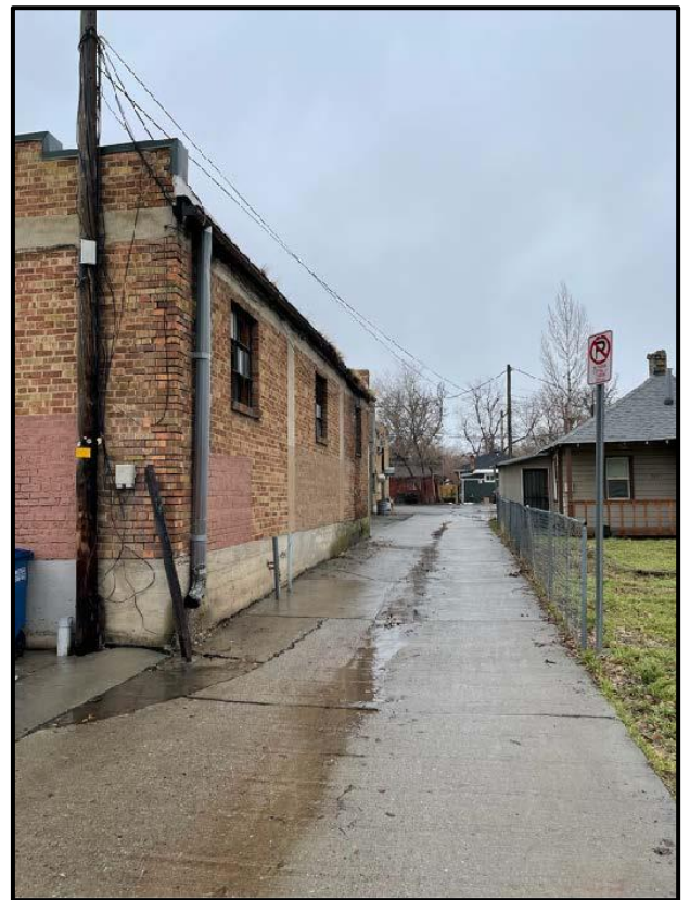
Grace Ct and portion of building to be demolished
