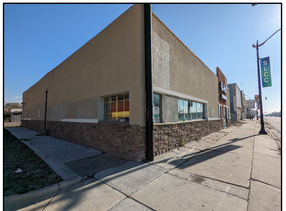
49 1791 S State St – to be demolished
