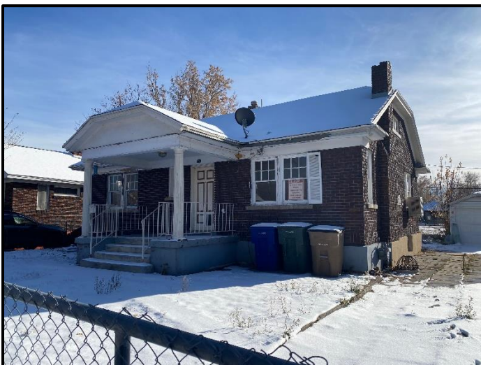
120 E Coatsville Ave, facing southeast
