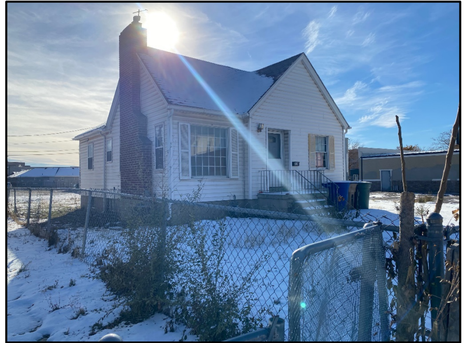
118 E Coatsville Ave – to be demolished
