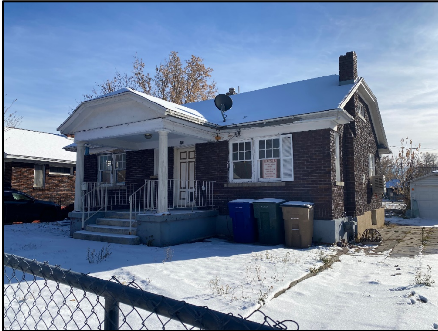
120 E Coatsville Ave – to be demolished
