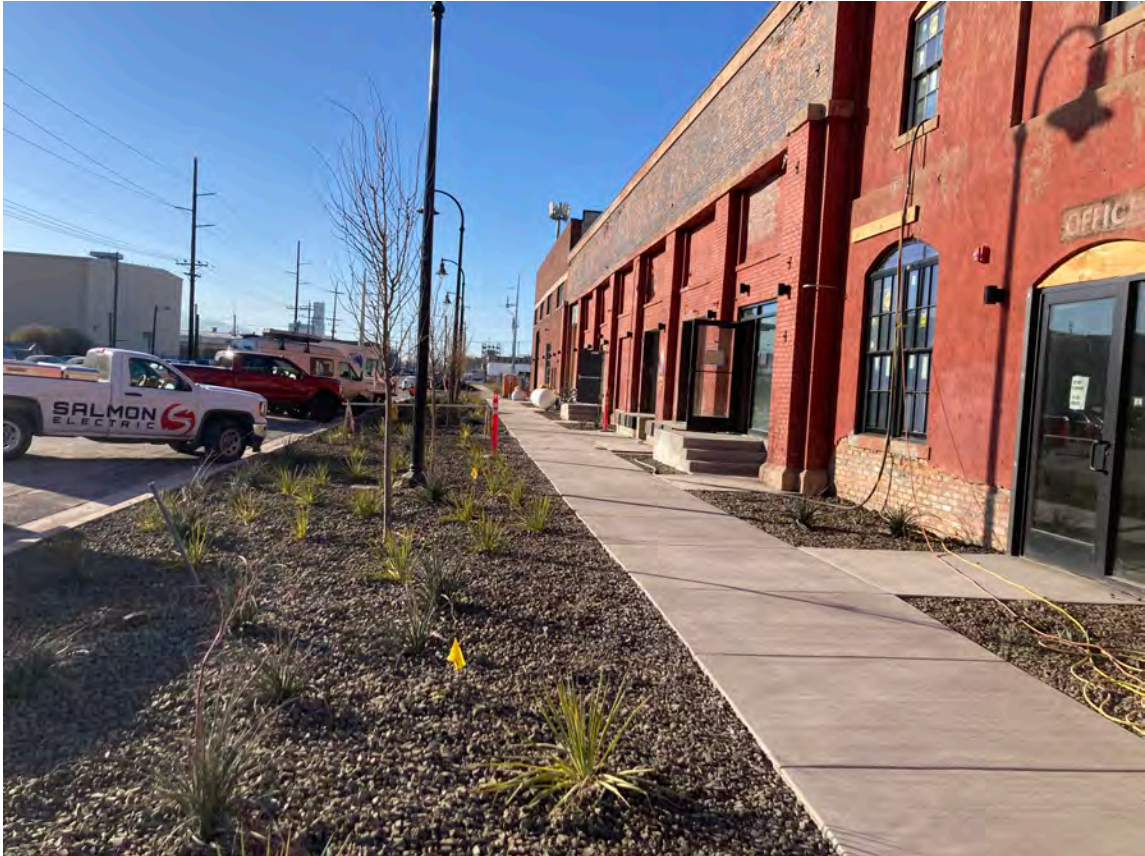
(Adjacent building with zero lot lines and no setbacks)
