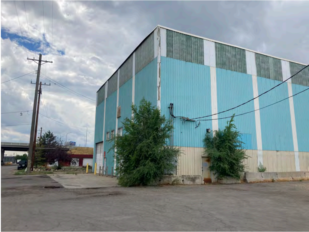
(Existing building on the West Village site with no front yard setback)
