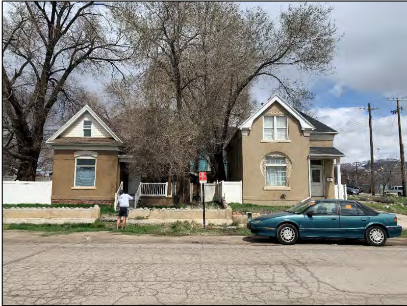
Two dwellings to be demolished on Fayette Avenue (looking north)
