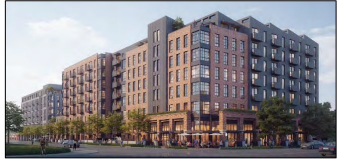
Building 3: Northeastern corner with ground floor retail on the corner of 400 W & 900 S
