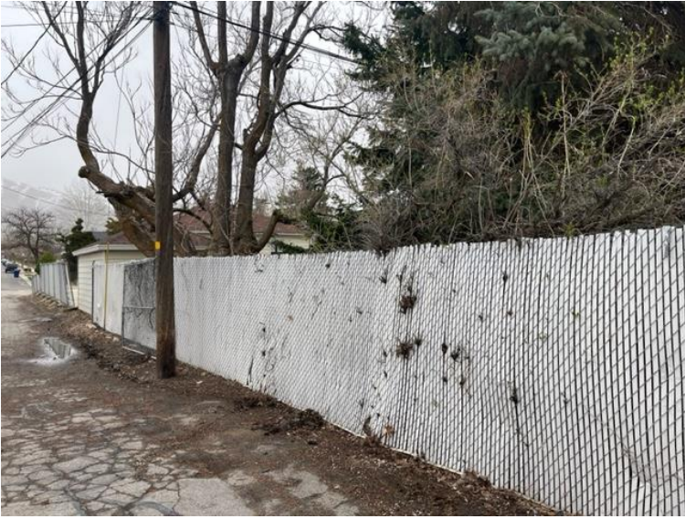
Photo of Looking Southeast
