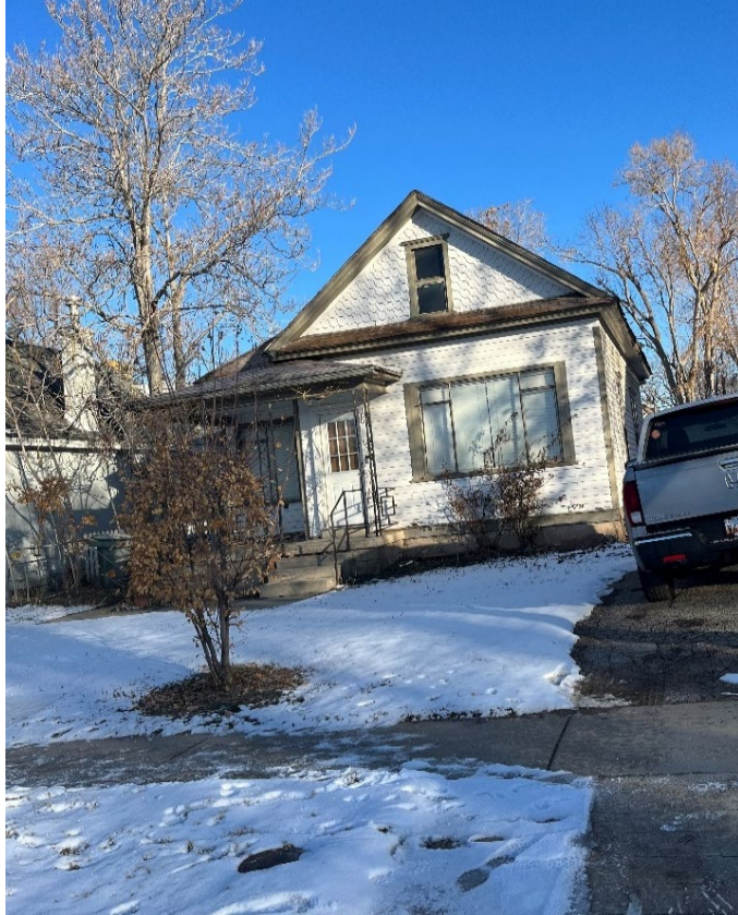
View of property from Princeton Ave (existing single family house to be demolished)
