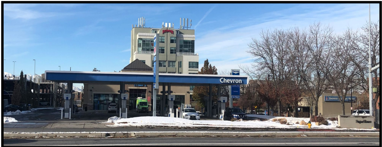
Chevron Gas Station and Convenience store located on the Southwest corner of 2100 S. 1300 E.
