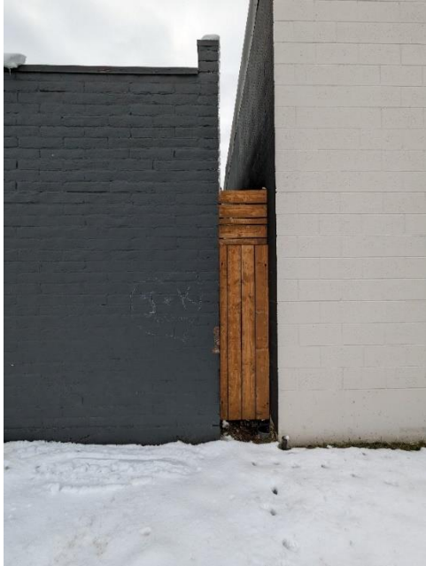
Existing space between adjacent property building to the west
