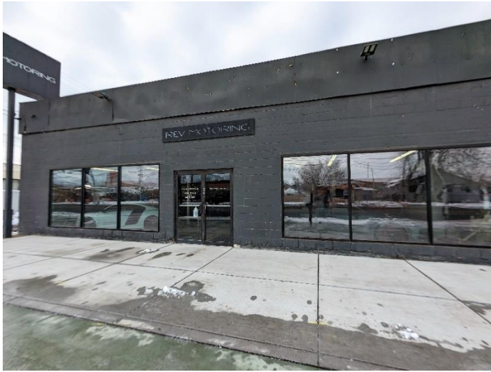
Front of existing building on 300 W
