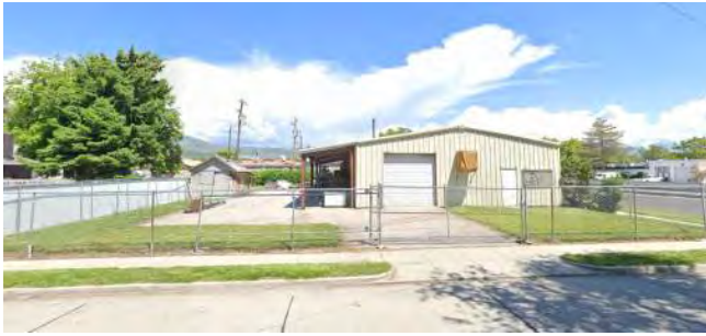
Existing warehouse at 938 W South Temple will be Removed
