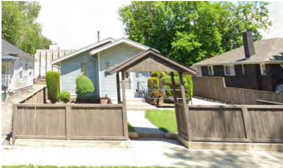
Existing House at 28 W Chicago St will be Removed
