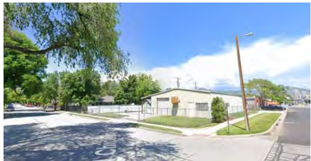
Looking North East at Site
