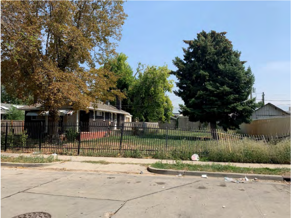
Existing dwelling at 18 N Chicago Street
