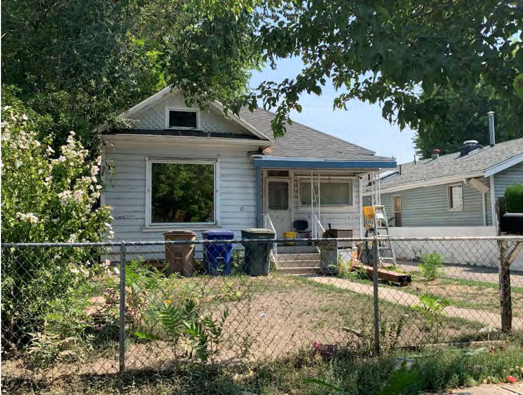
Existing dwelling at 30 N Chicago Street
