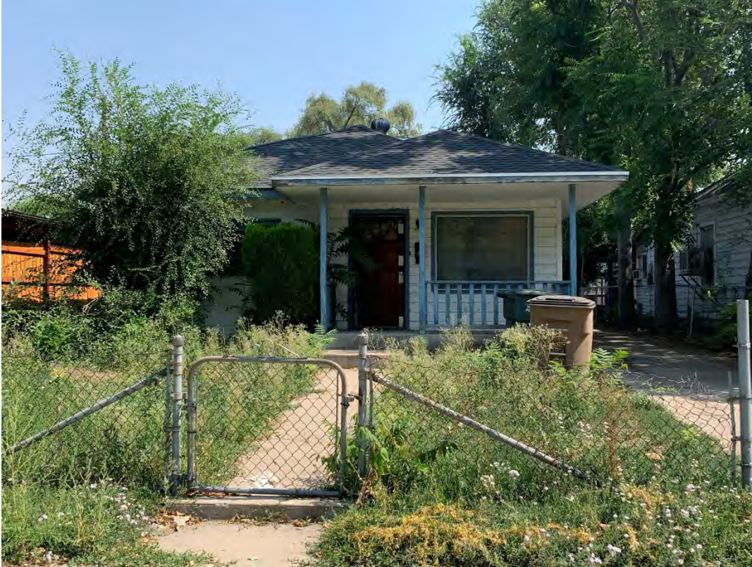
Existing dwelling at 36 N Chicago Street
