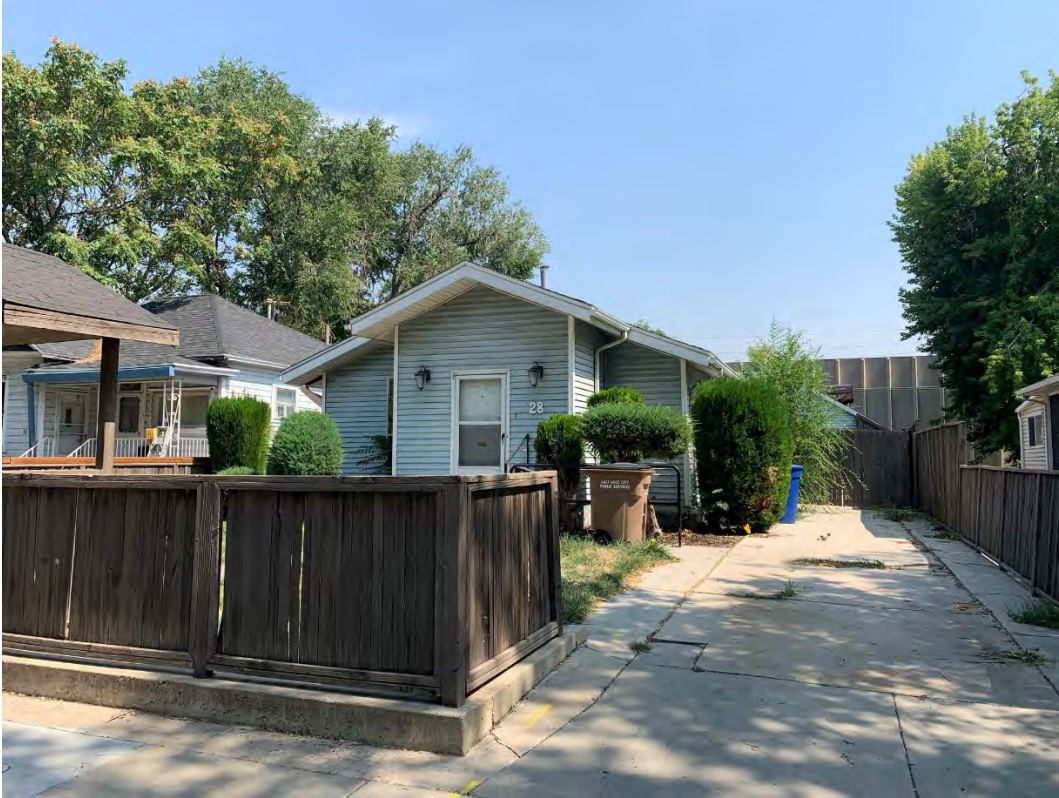
Existing dwelling at 28 N Chicago Street
