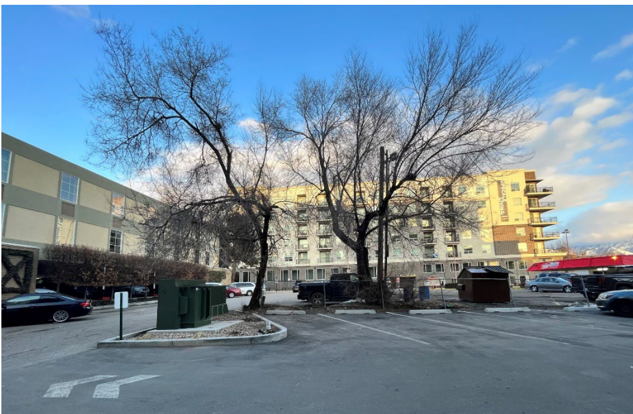
352 Denver St (left) and Encore Apartments from Starbucks parking lot
