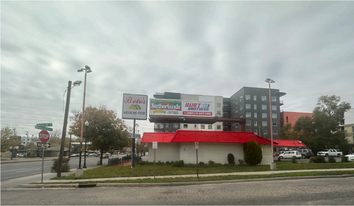
Single-story restaurant on corner of 400 S & Denver St.
