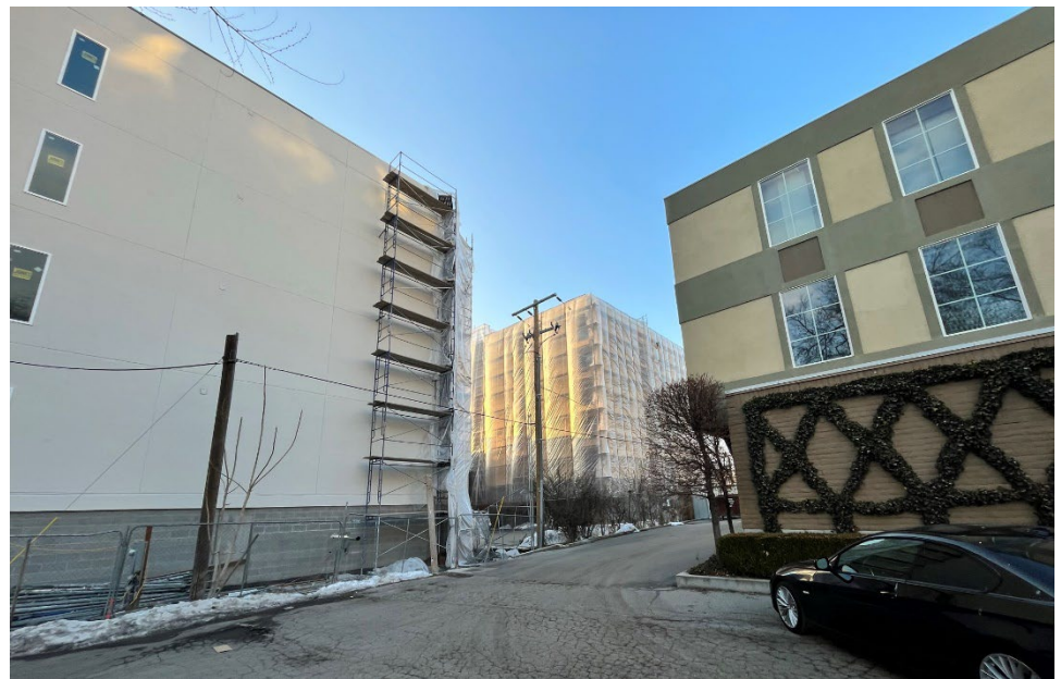
Aqui 355 (left), TAG 343 (middle), and 352 Denver St (left) from Beto's parking lot
