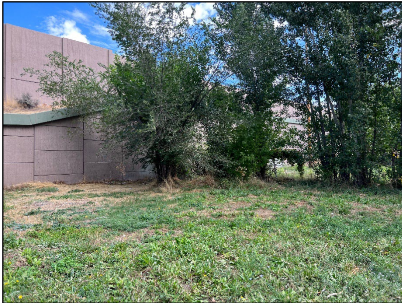
Subject Property – Looking northeast at I-80 sound wall
