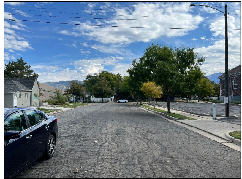
Warnock Avenue as viewed from east side of subject property
