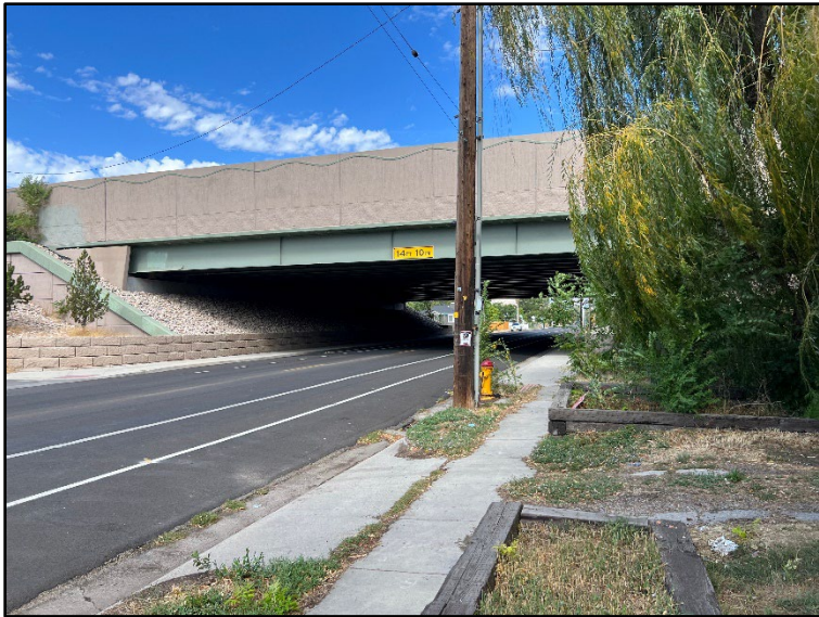
Looking north from subject property at I-80 overpass of 500 East
