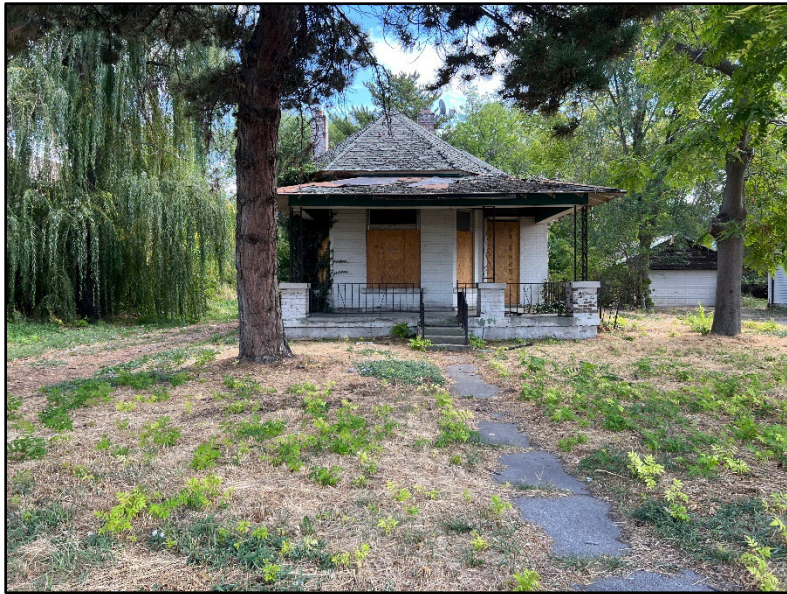
Subject Property – Looking east from 500 East
