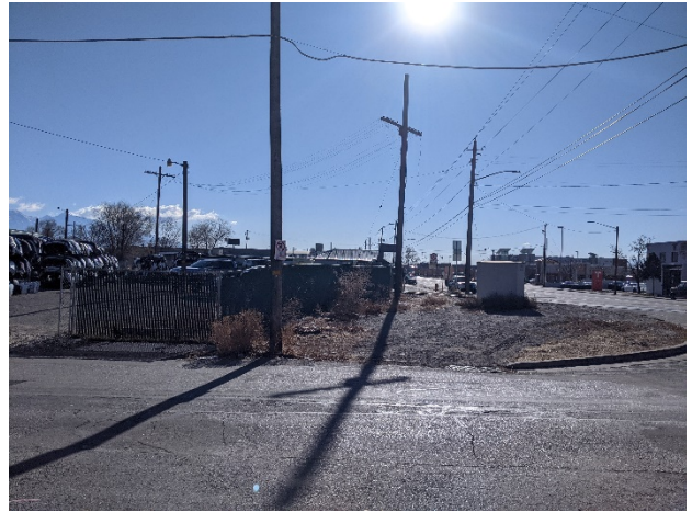
Figure 7 – Northwest corner of the property where it the new sidewalk will connect to the UTA's abandoned rail line
