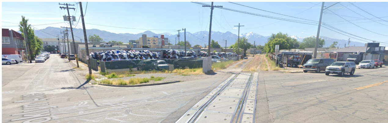
Figure 14 – 269 W Brooklyn and the UTA's abandoned rail line seen from the intersection between Brooklyn Avenue and 300 W
