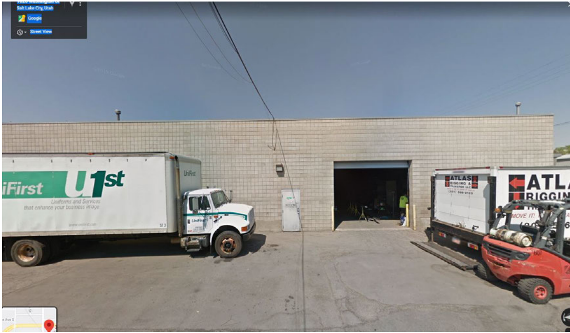
Building at South West Corner of Brooklyn & Washington, Washington Facade
