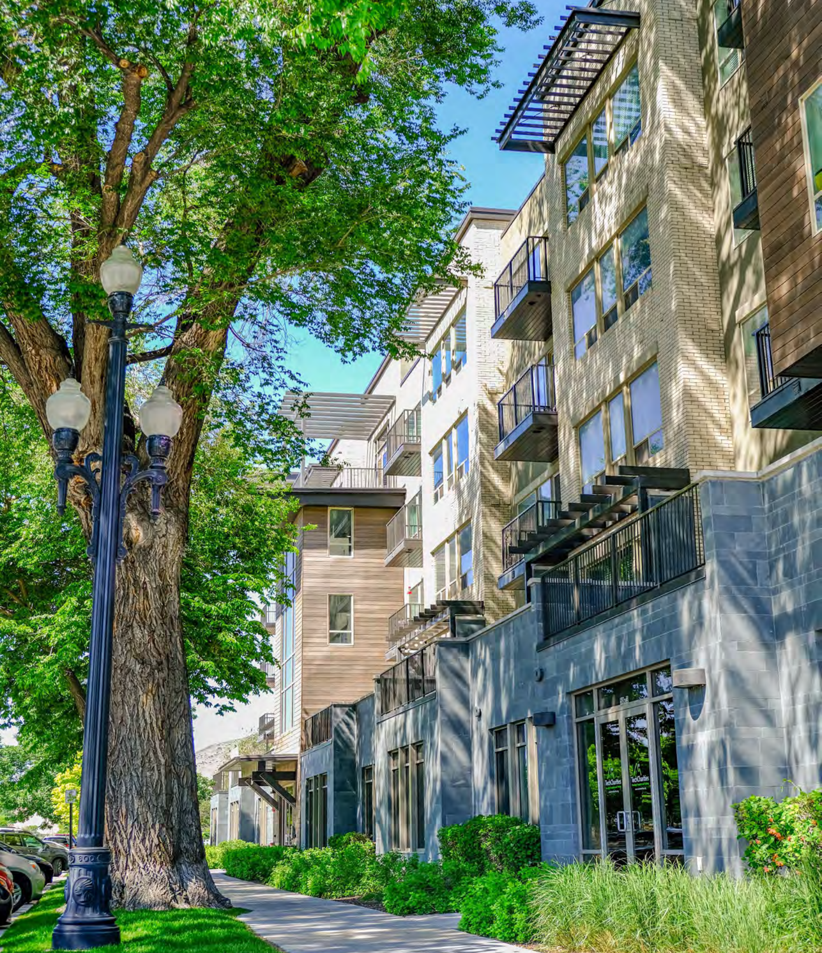
When planted to cast shade on building windows and sidewalks, trees reduce energy use and cool pavements
