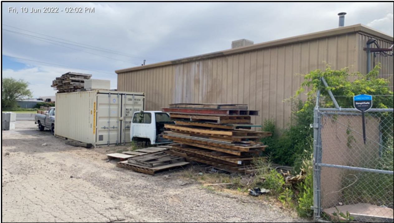
Subject property, facing southwest. Storage outside of the container will need to be screened or relocated.
