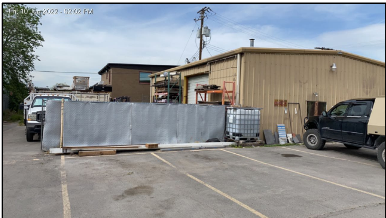
Outdoor storage may be permitted behind this fence. The storage of items higher than the height of the fence must be screened.
