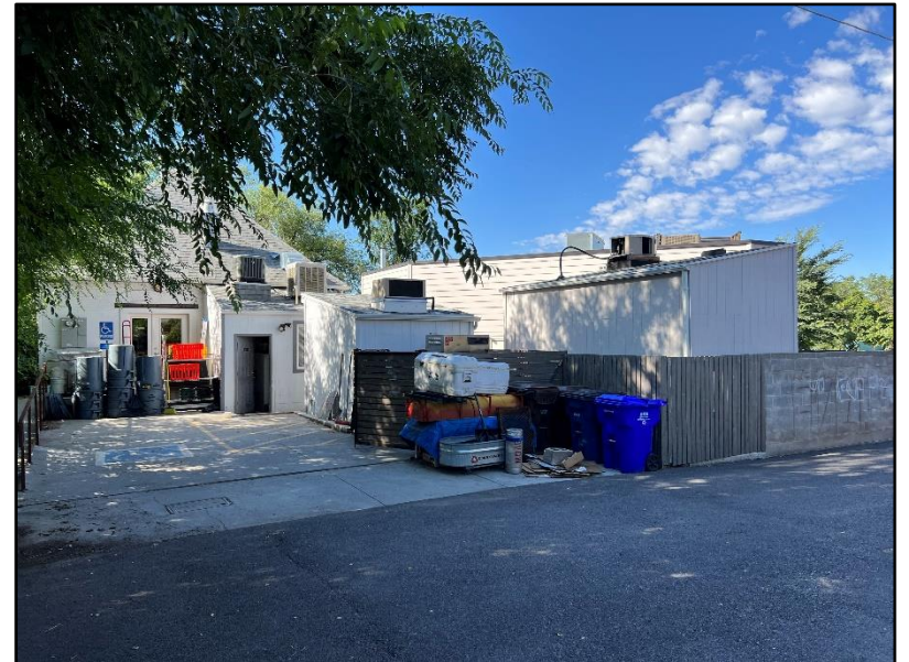
ADA parking stall for adjacent business is accessed through shared right of way with subject property
