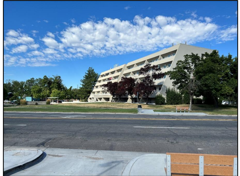
West side of 500 E as viewed from subject property
