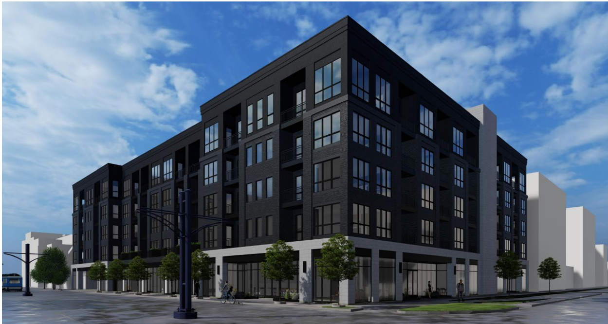
Final rendering of 200 W façade with staff's concerns taken into consideration. Changes were made to the colors, proposed materials, and ground floor glazing to create three distinct building masses along 200 W.
