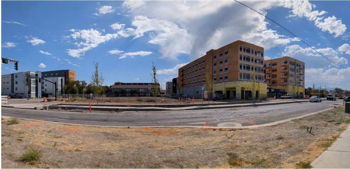
Existing conditions from 900 S looking south. The Urban Alfandre project is under construction to the right.
