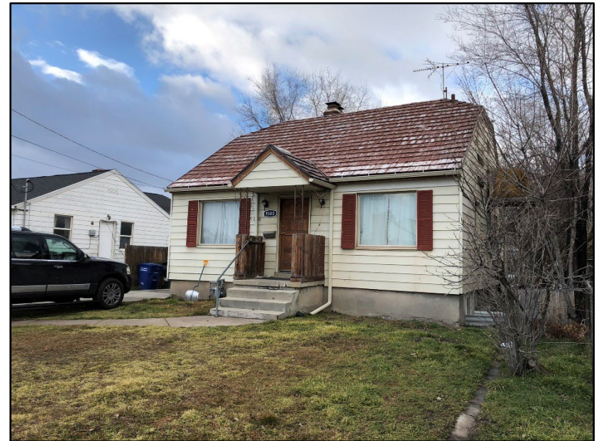
Subject Property – 1500 W 500 North
