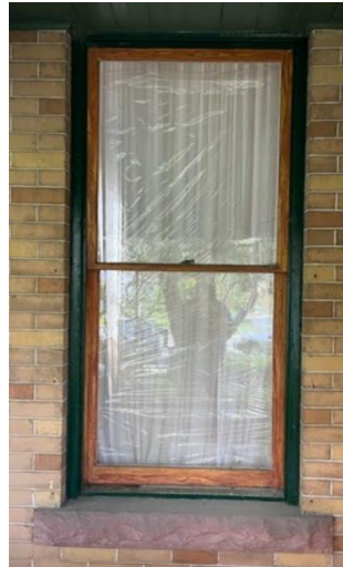
Photo of Eastern Most Window on North Elevation
