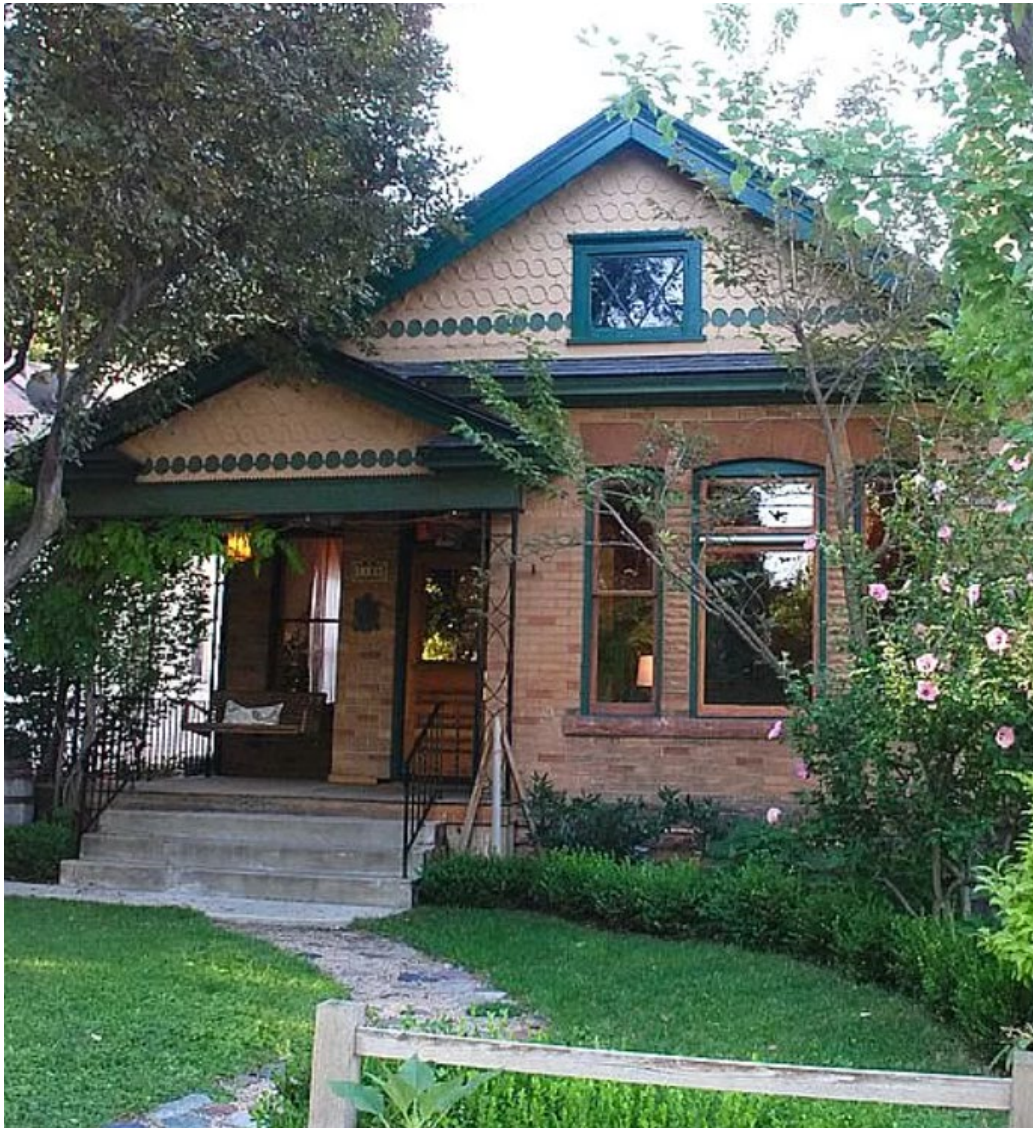
Photo of Front Elevation (North) Photo from Zillow, c. 2020
