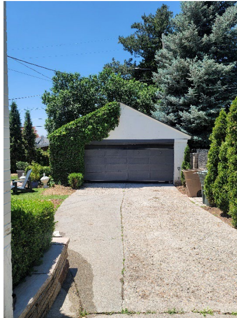
View of existing detached, accessory structure
