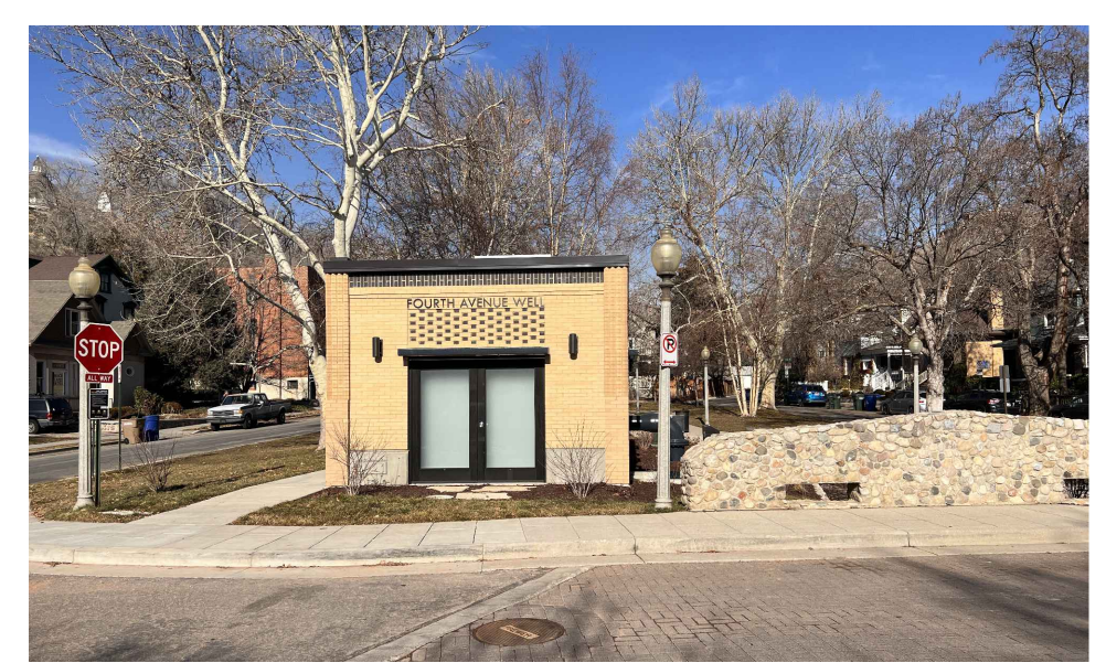
9 FOURTH AVENUE WELL ELEVATION FACING FOURTH AVENUE
