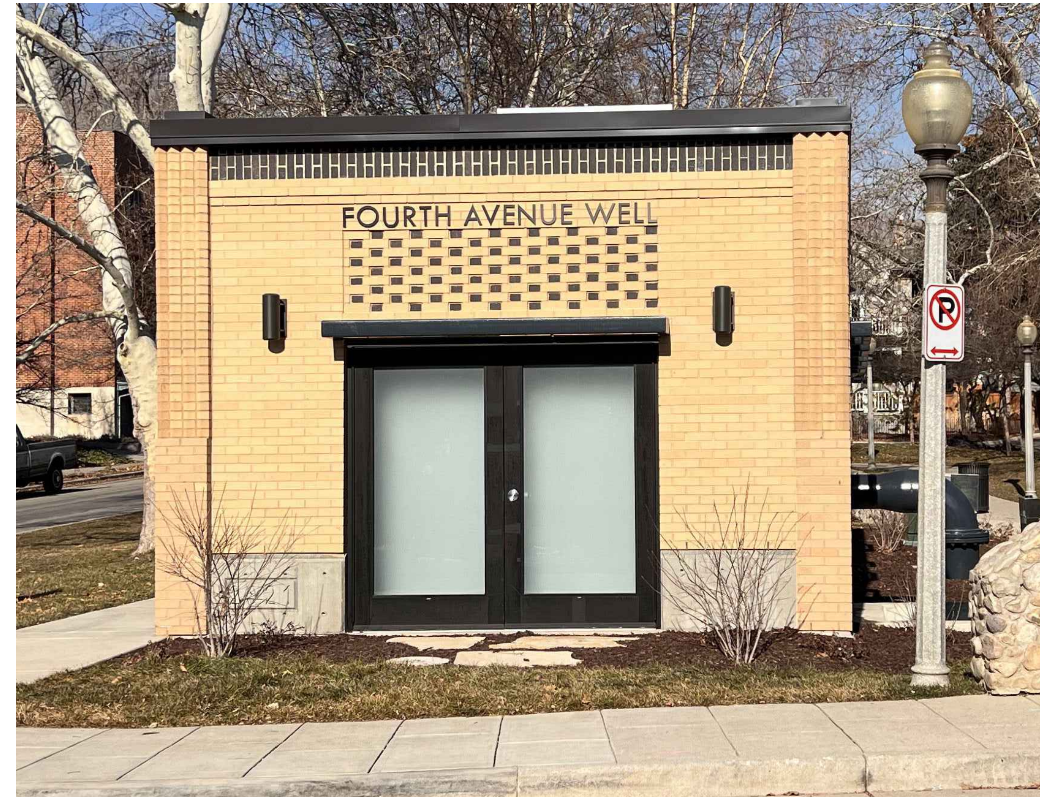
EXAMPLE OF LIGHT COLORED BRICK DARK STEEL OVERHANG DARK METAL DOORS WITH OBSCURED GLASS CONCRETE BASE
