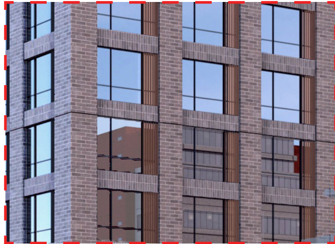
EXTERIOR WALL A
