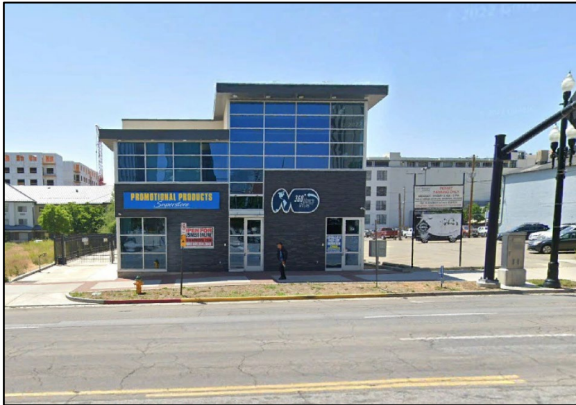
Adjacent Commercial Building to the North
