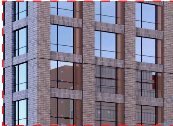
EXTERIOR WALL A
