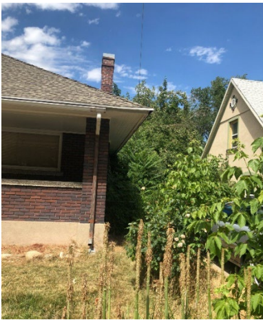
North property line -four feet from dwelling to property line
