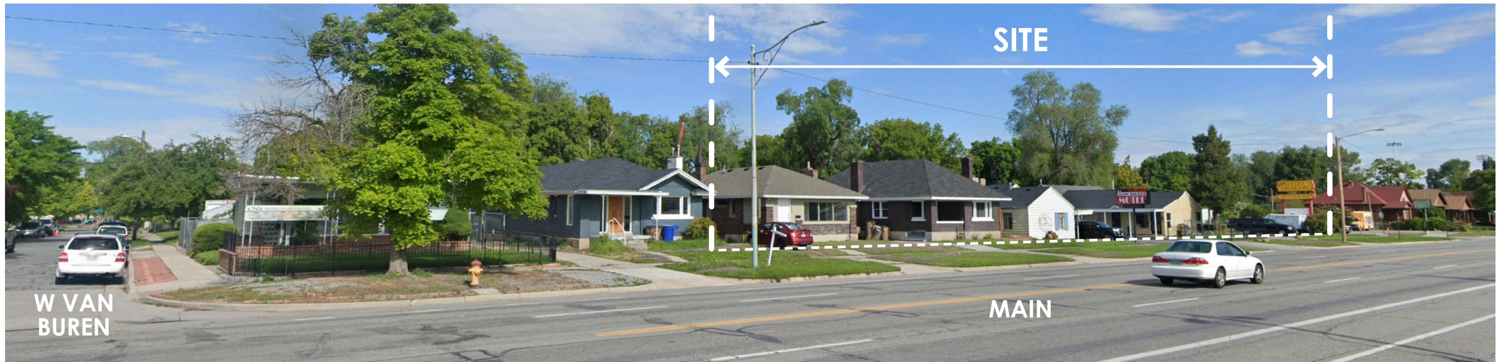
MAIN ST. @ VAN BUREN LOOKING NW
