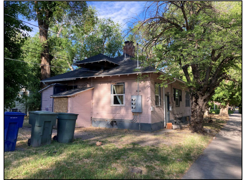
Subject Property – Duplex 1 – Back view
