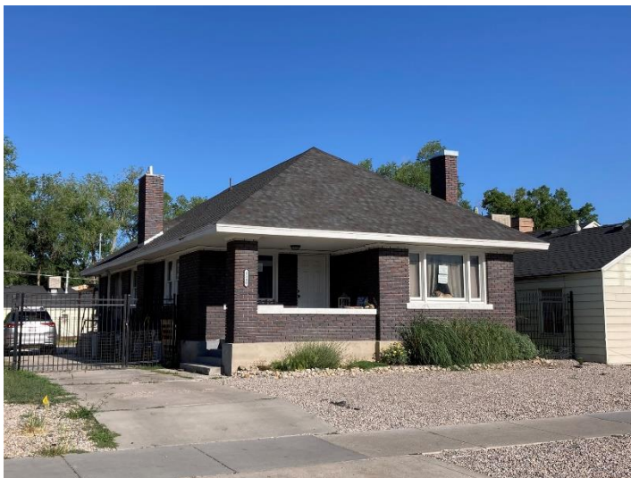
Existing dwelling at 1540 S Main – to be removed
