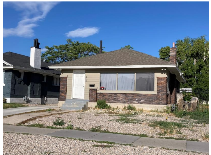
Existing dwelling at 1546 S Main – to be removed
