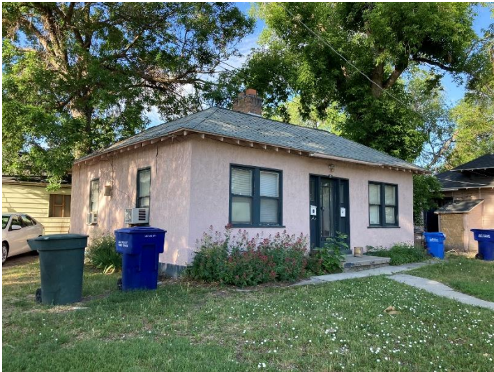
Existing duplex at 1515 S Richards – 1 of 2 duplexes
