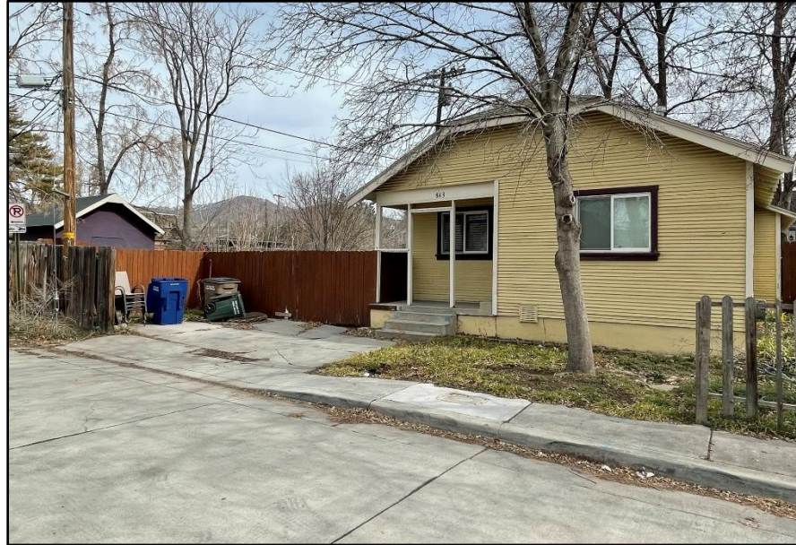
Area of future access from Lake Street
