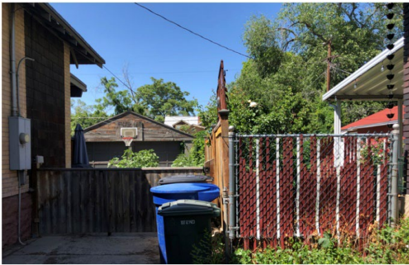
View of back driveway area – garage to be removed
