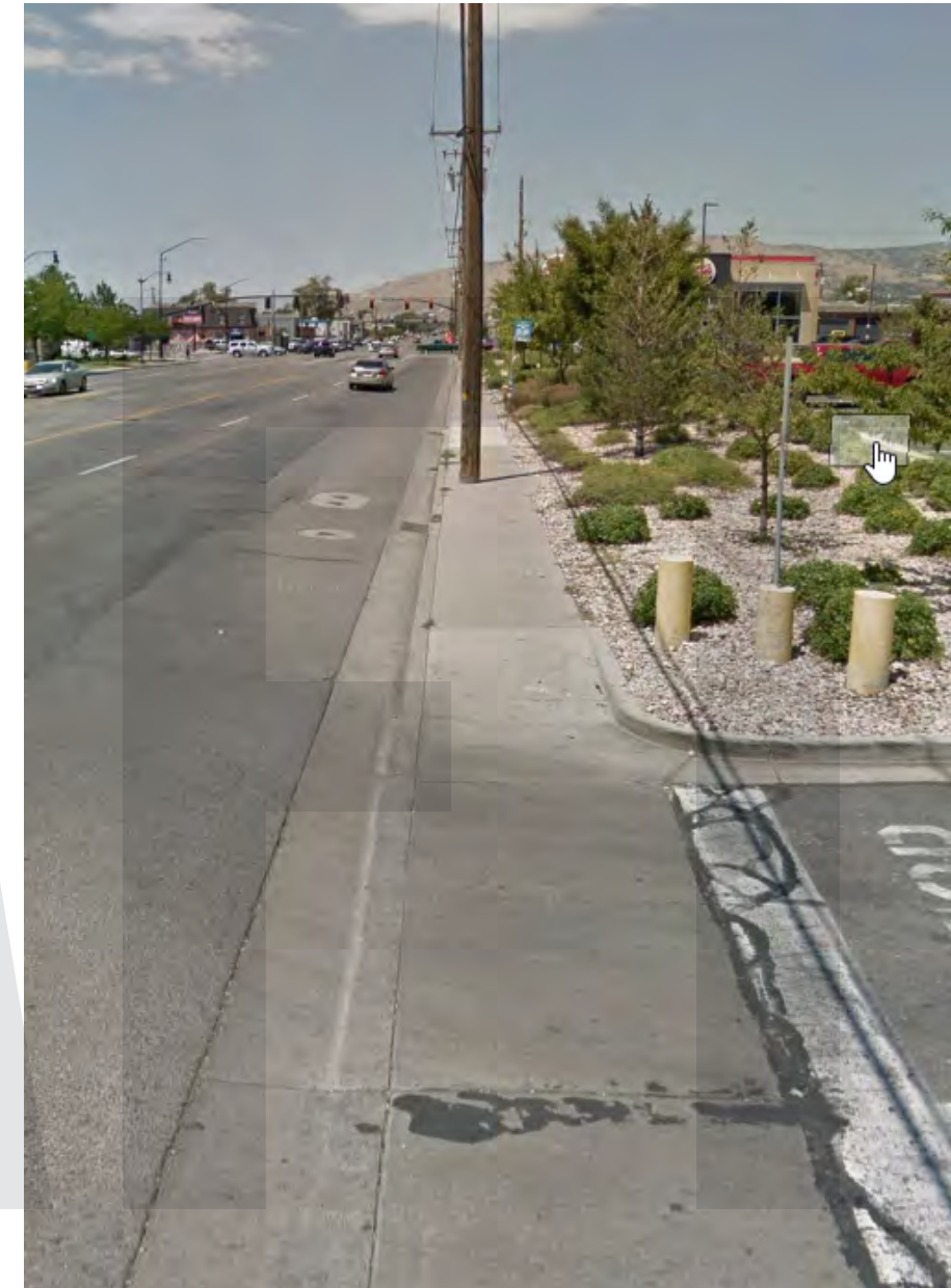
Figure 29 - Narrow Sidewalk with Obstructions along 300 West
