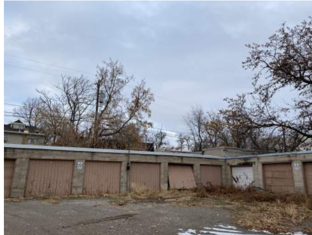
Storage garages at interior of site, along North property line.
