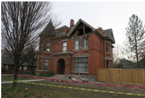
Figure 2: Photograph of damage to Sears Mansion following March 2020 earthquake.
