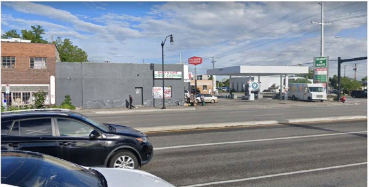
Looking West, across the street - several parcels with a variety of land uses such as retail, restaurants and a gas station zoned CC
