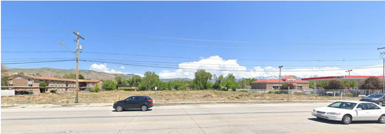
Existing site at 750 N Redwood Rd.
