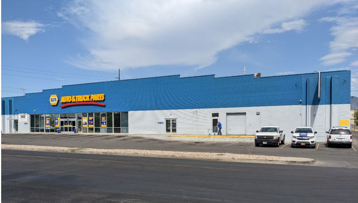
Auto parts store located across the street to the east of subject property-zoned M-1
