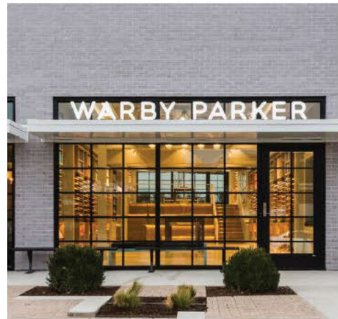
LIGHT GRAY COLOR MODULAR BRICK MASONRY OVER PAINTED STOREFRONT
