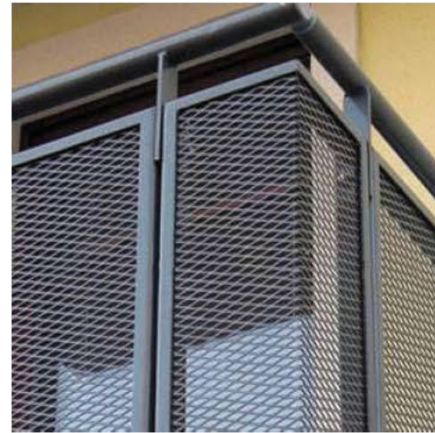
PAINTED STEEL C-CHANNEL SUPPORT AT BALCONY PERIMETER WITH MESH PANEL GUARDRAIL
