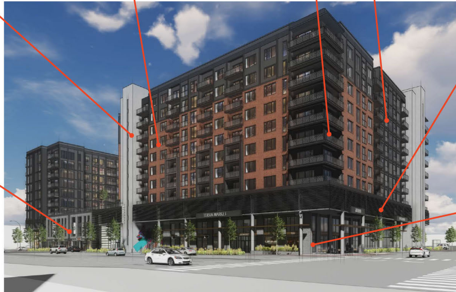
PAINTED STEEL C-CHANNEL SUPPORT AT BALCONY PERIMETER WITH MESH PANEL GUARDRAIL
