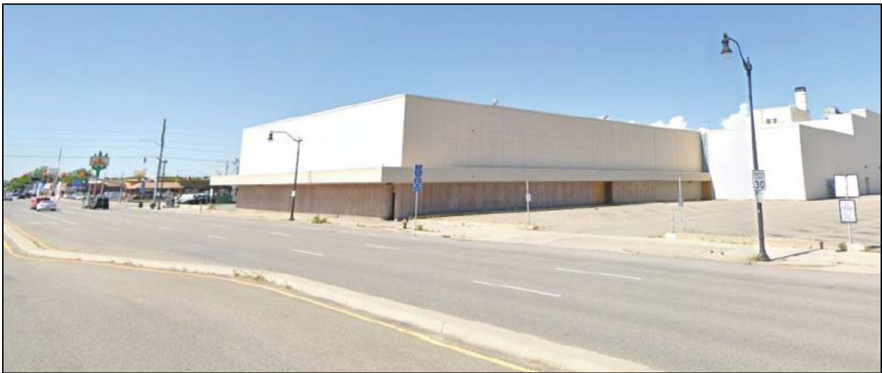
View of Site, North/East Perspective from State Street
