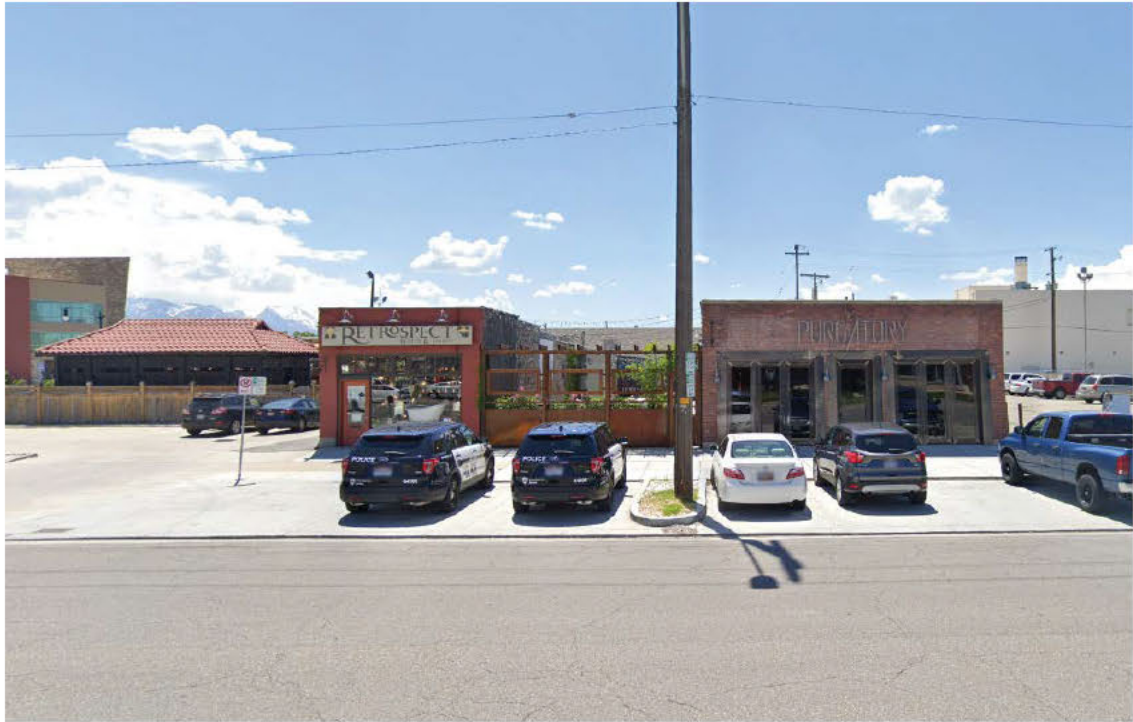
E 700 LOOKING SOUTH
