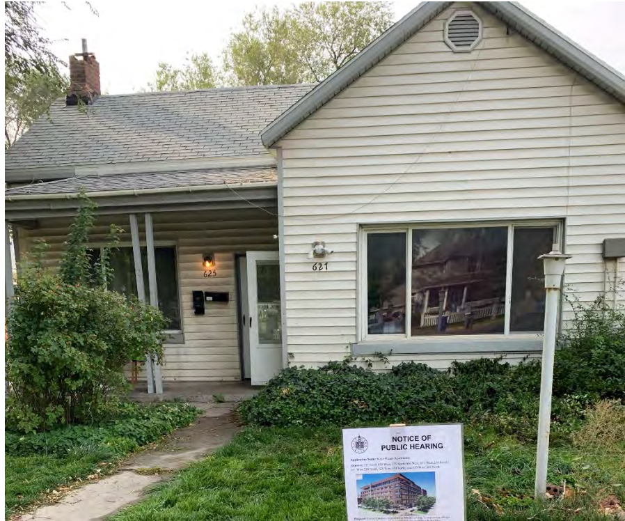
Figure 7: 625 West 200 North, currently a single-family dwelling
