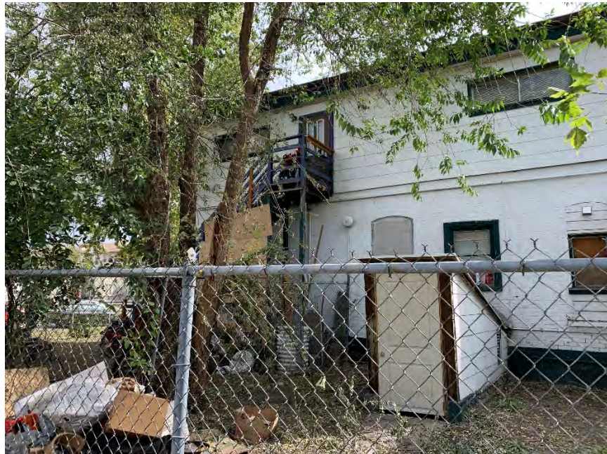
Figure 12: 175 North 600 West, currently multi-family dwelling
