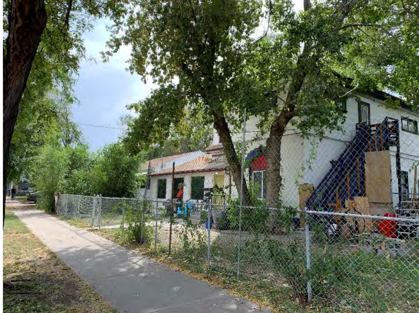
Figure 11: 175 North 600 West, currently multi-family dwelling
