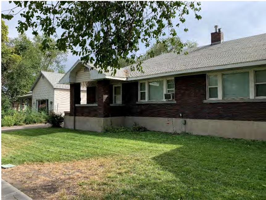
Figure 6: 633 West 200 North - currently a two-family dwelling
