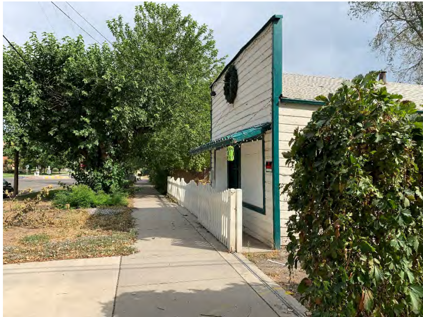
Figure 10: 613 West 200 North, view of "shop" from 200 North
