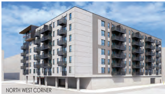
NORTH WEST CORNER
