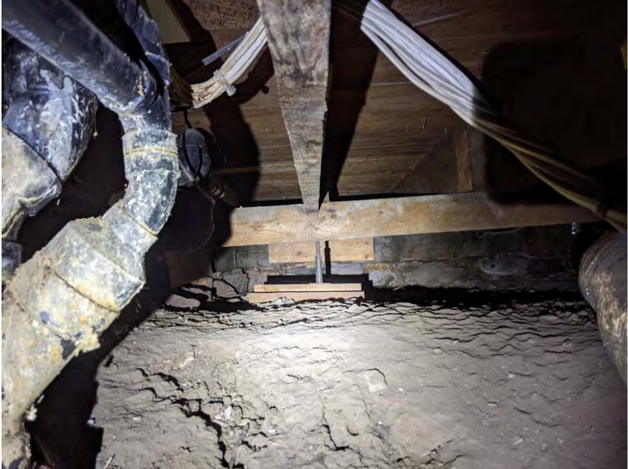
More leveling / support jacks.
