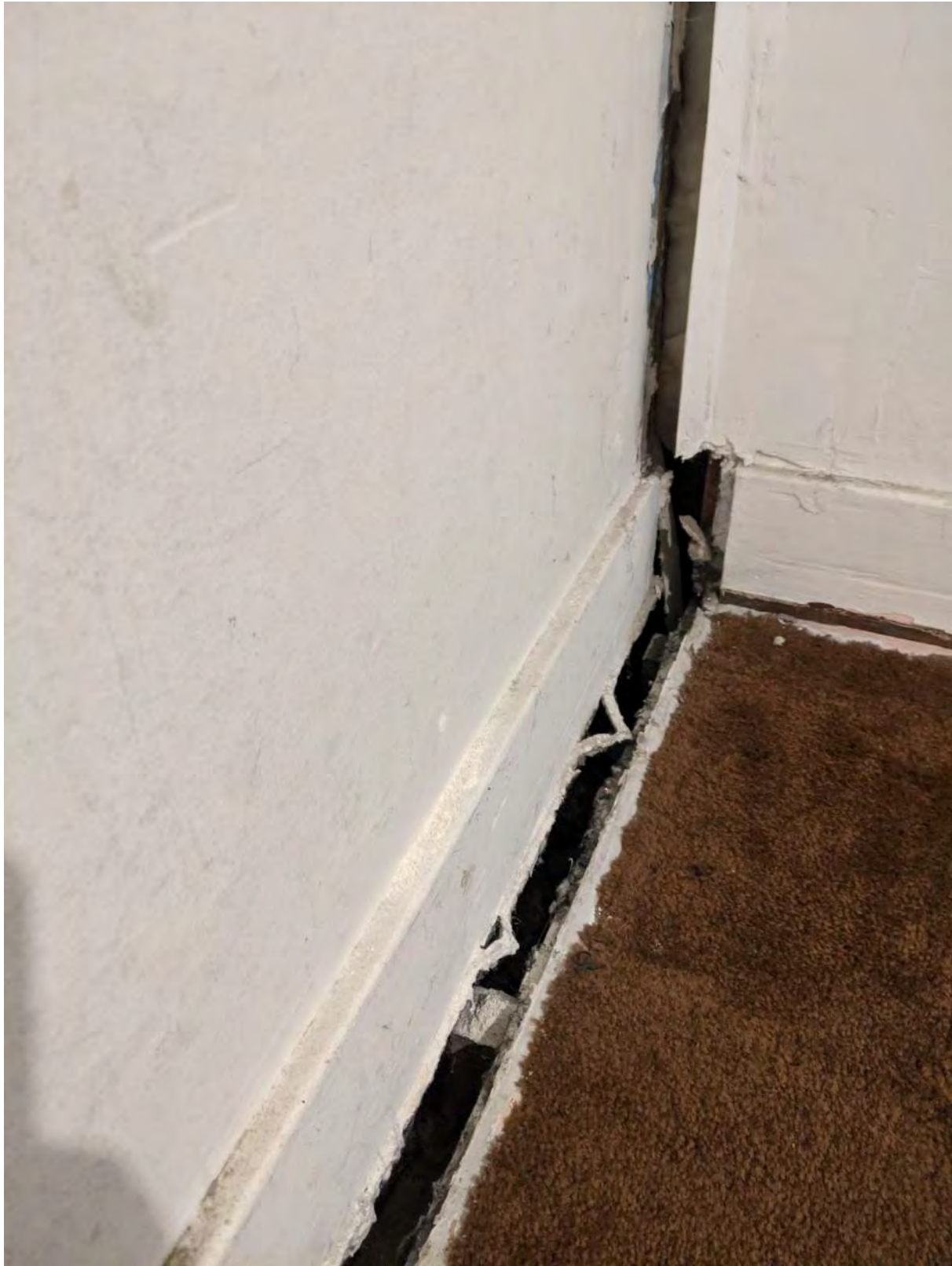
Continuation of Floor and Wall separation in the Bedroom
