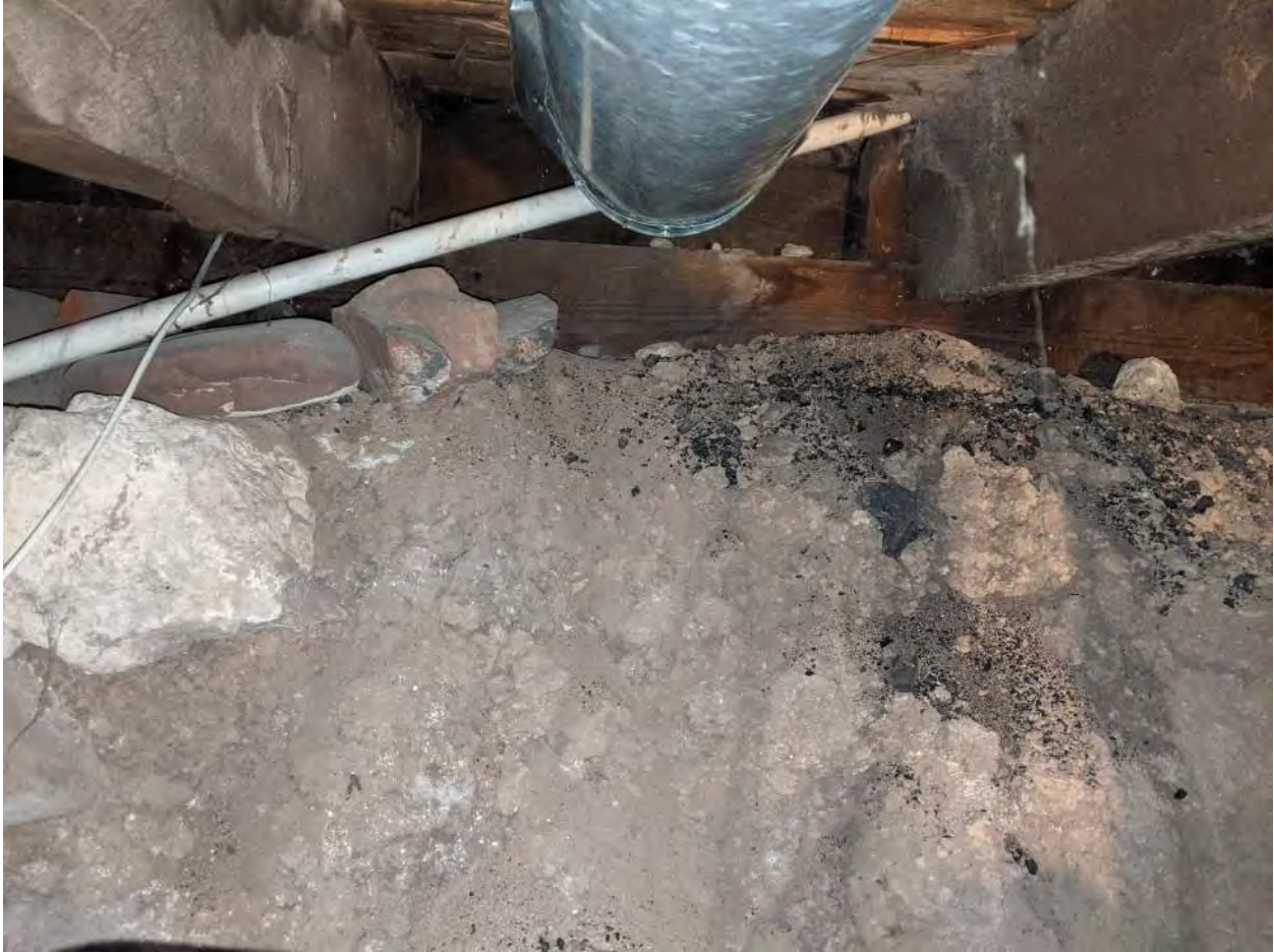
Typical wood foundation perimeter joist bearing on earth.
