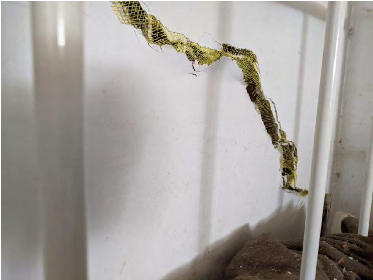
North West corner close up Living room.
