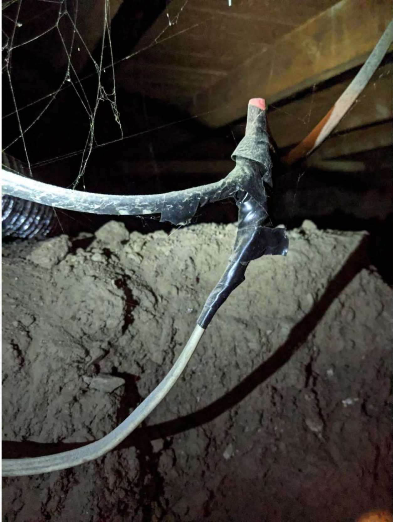
Typical wiring connection with ungrounded wire.
