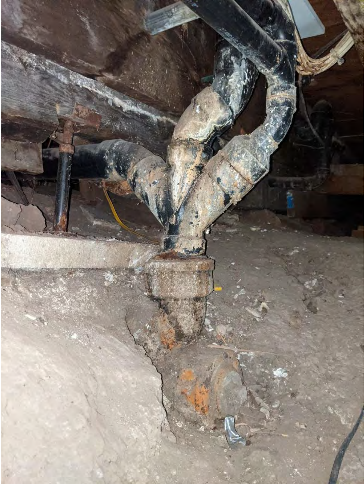
Typical leveling jack placed on paver, bearing over sewer line.
