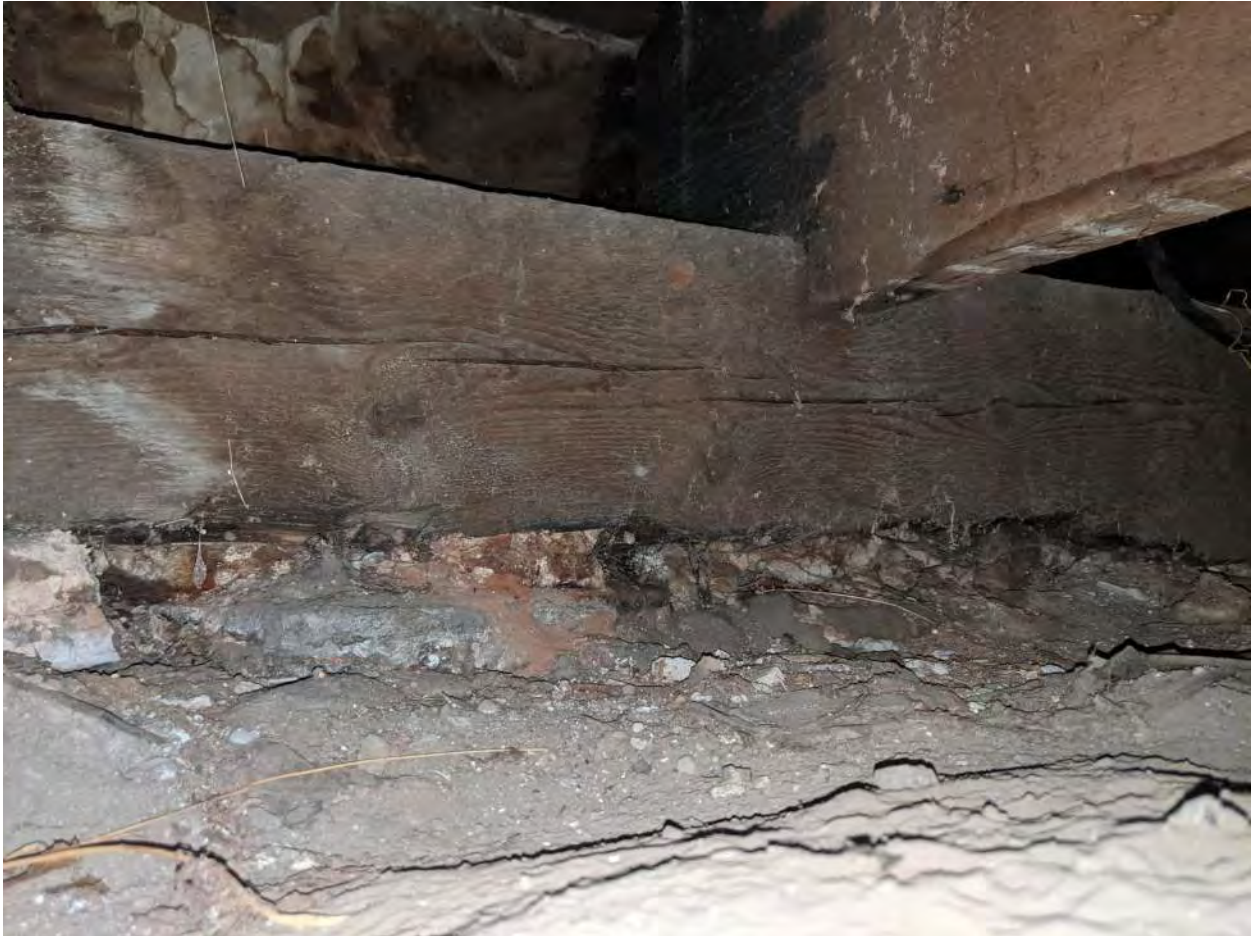
Typical South East foundation. Wood bearing on earth.
