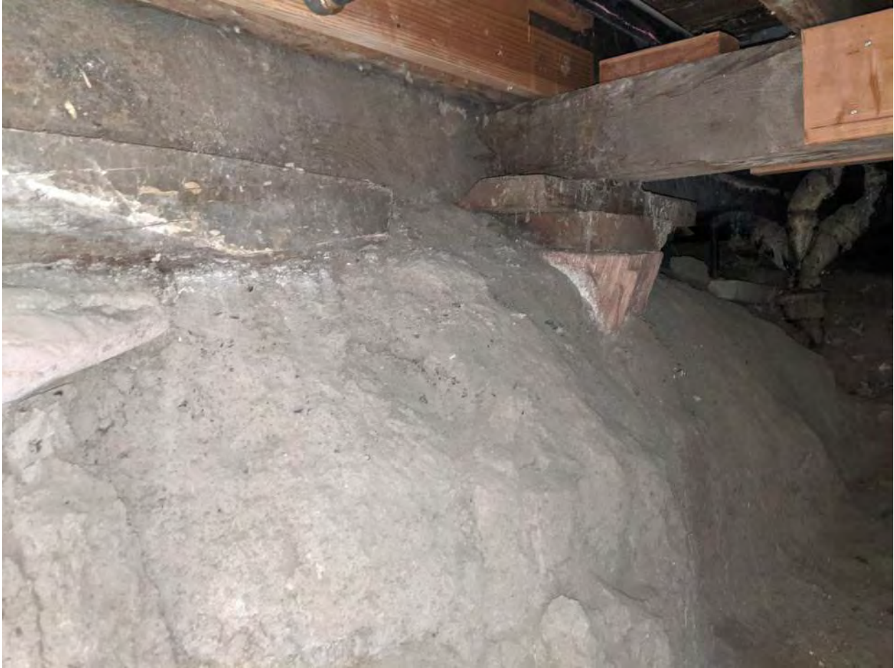
South foundation wall. No reinforcements present.
