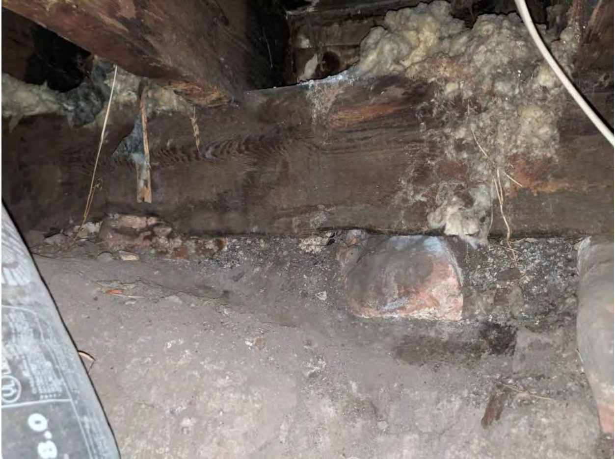
North East foundation, typical of entire foundation.
