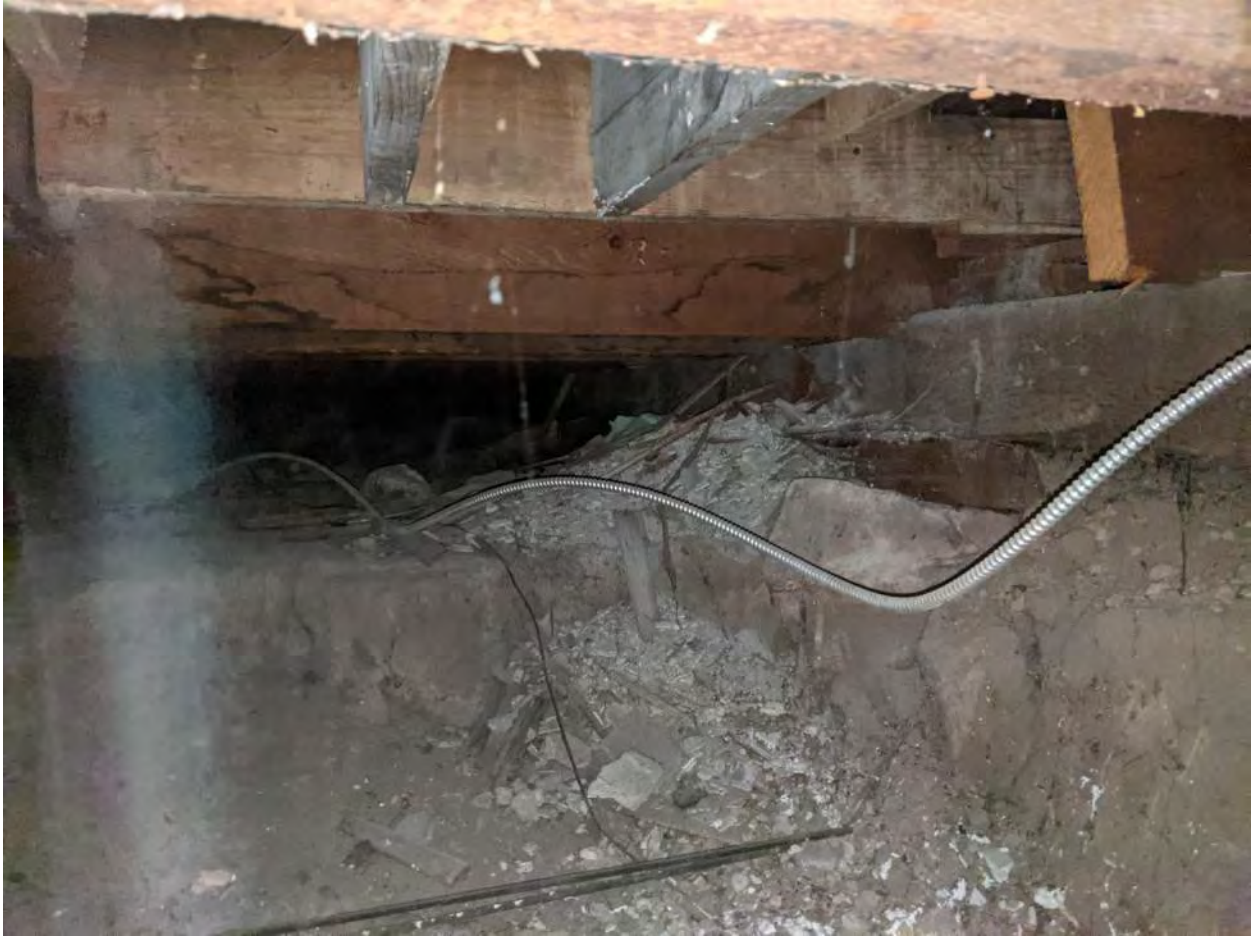
Eastern foundation on earth.
