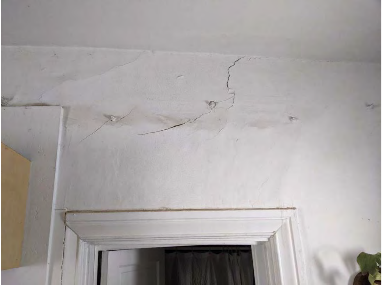
Bathroom roof joist anchors pulling away from wall.
