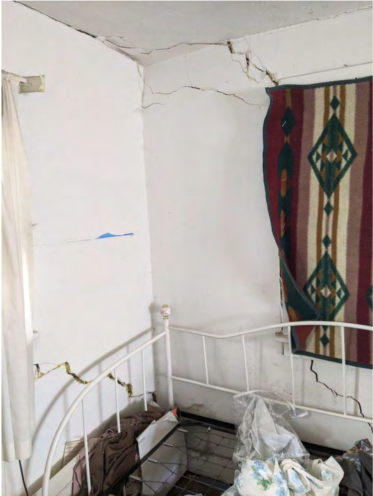
Interior of North West corner
