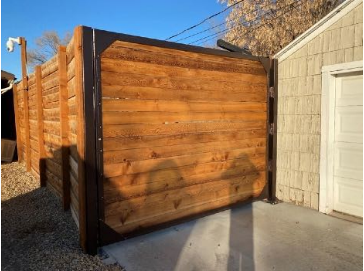
Powder coated steel gate frame with cedar planks run East to West at South West corner of fence on west property line.
