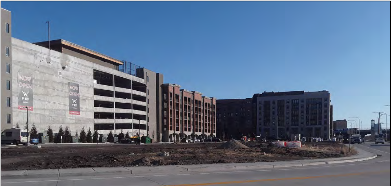
View of Site, looking south on 490 West
