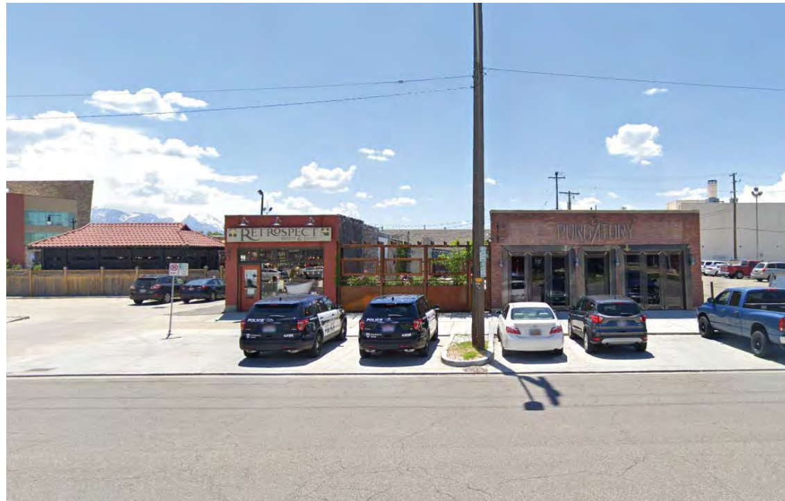
E 700 LOOKING SOUTH
