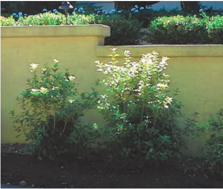
Capped, concrete retaining walls
