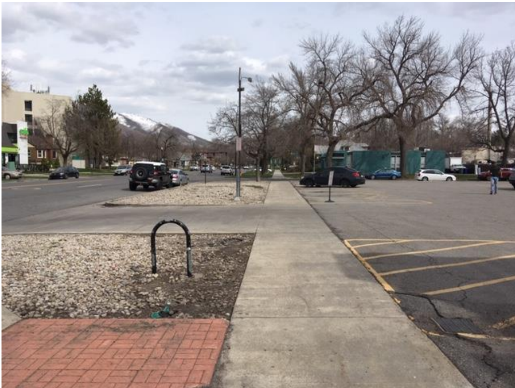
Park strip in front of the subject properties
