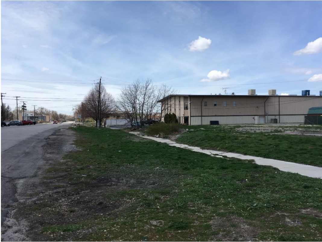
Street view of front of parcel looking west along 400 N.
