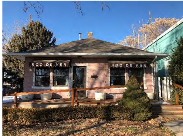
Existing structure with residential exterior to be demolished. New addition to Hip & Humble is proposed.
