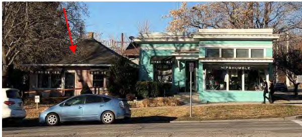
Existing structure identified with red arrow to be demolished and replaced with a new addition to Hip & Humble building
