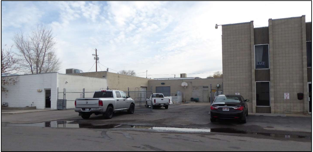
Image 5. Light Industrial Use Across the Street from Subject Property.
