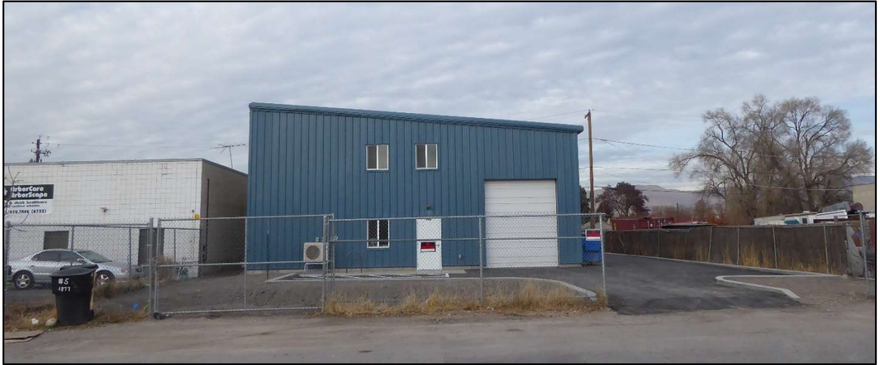
Image 1. Front View of Subject Property
