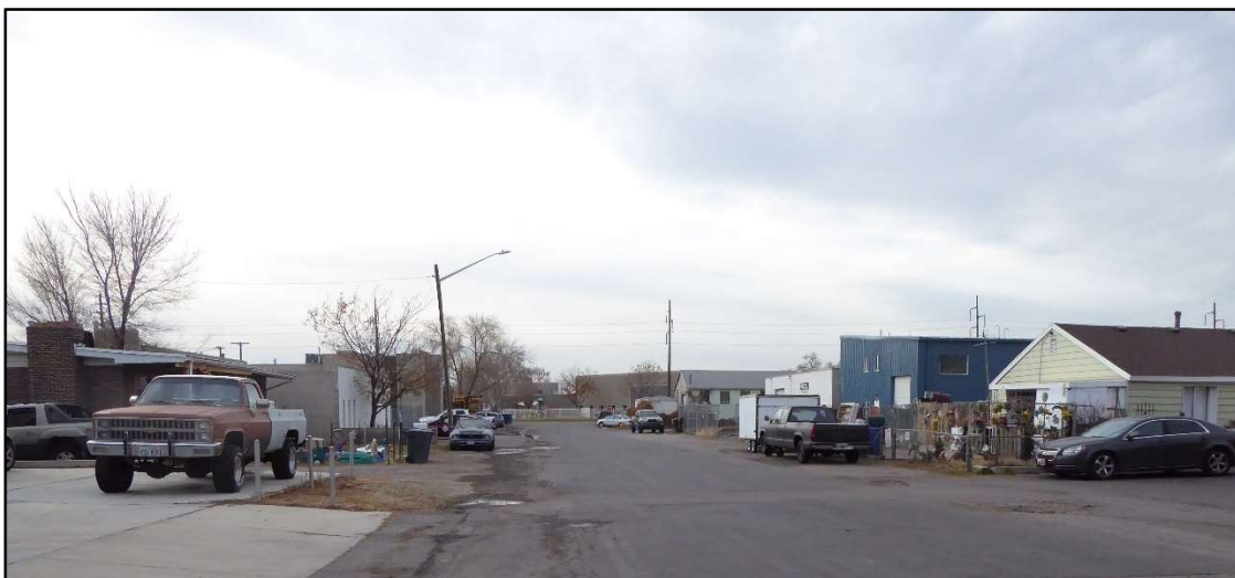
Figure 6. View of 1355 South Facing West (subject property is the blue building on the right)
