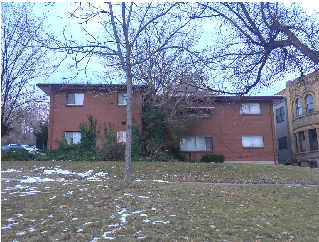
View of the property to the east and across 900 E
