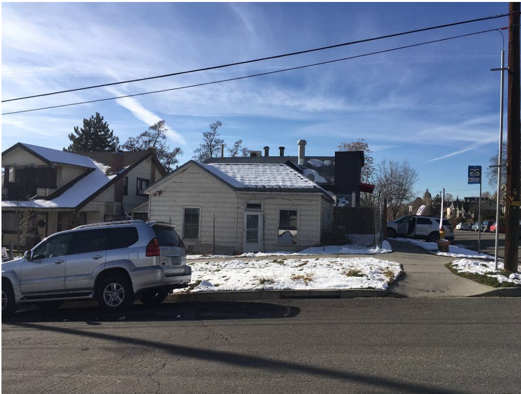
View of the subject property from G Street
