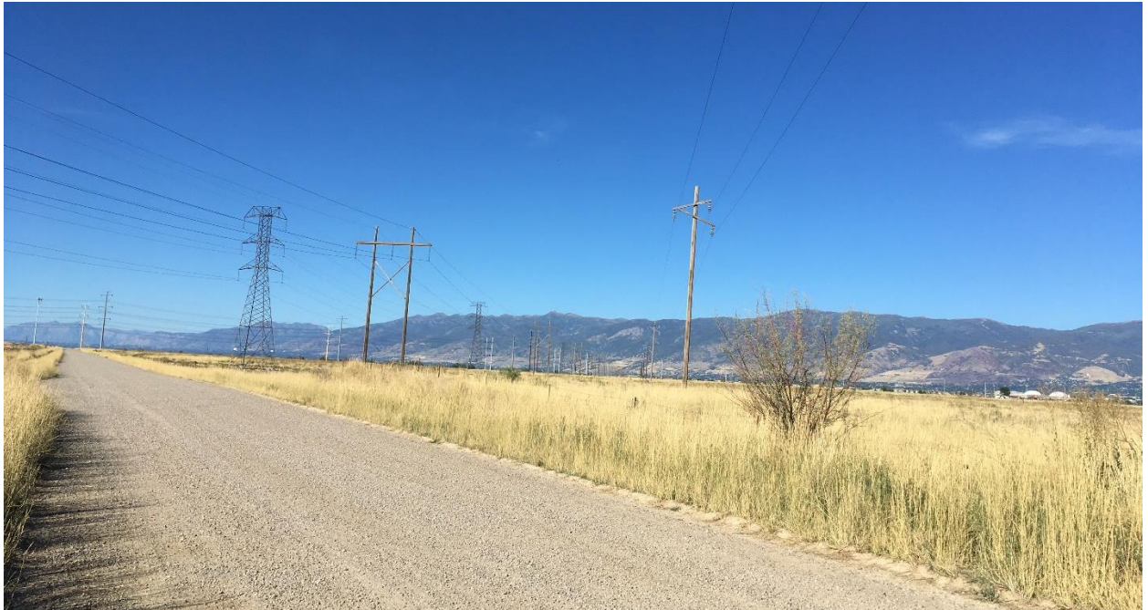
View of the power line corridor that runs north-east through the site (looking north-east into the site)
