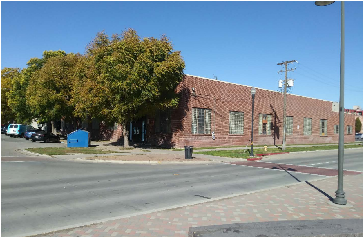
Building on the northwest corner of 300 South and 500 West
