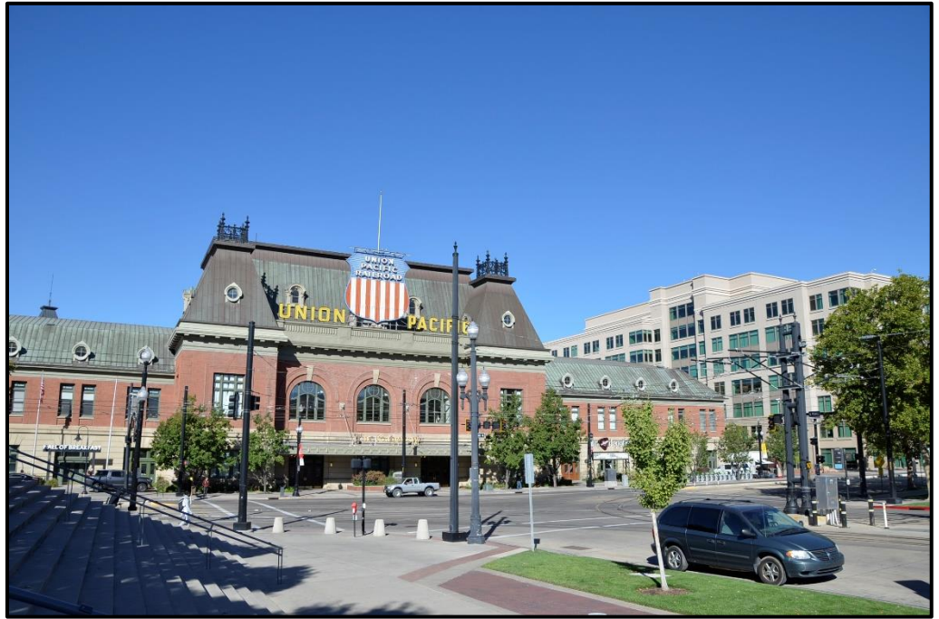
Front façade of the Union Pacific Train Station
