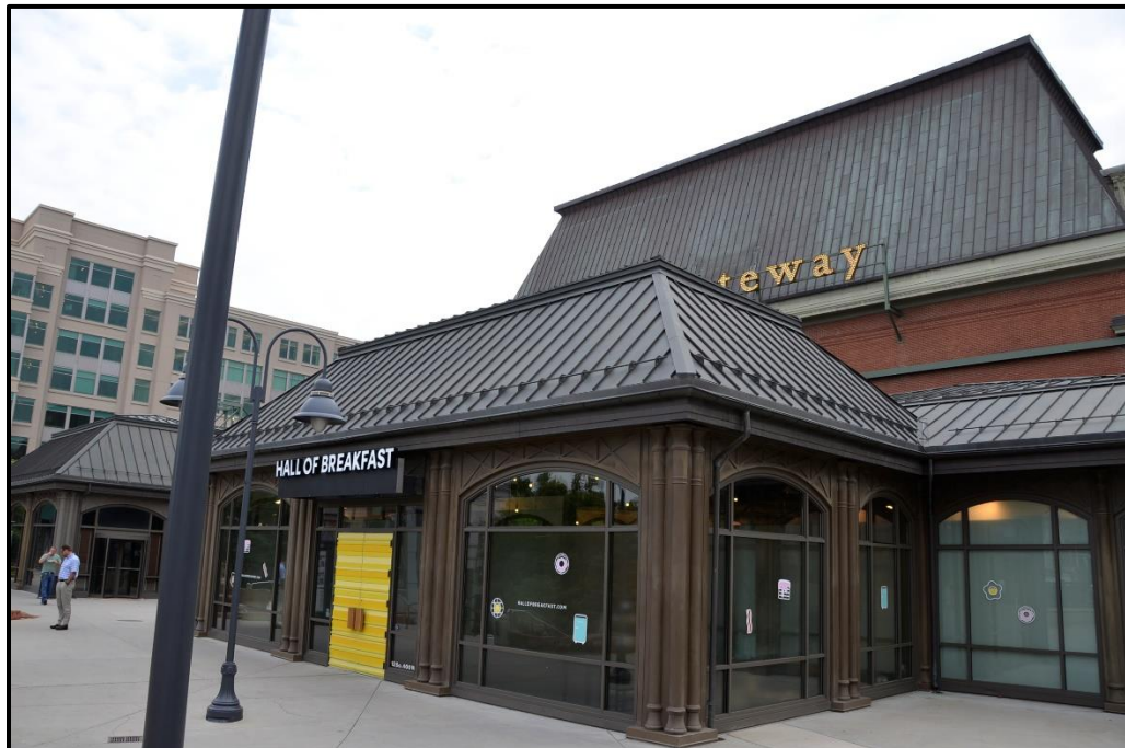
Existing 1-story buildings to be removed on the site
