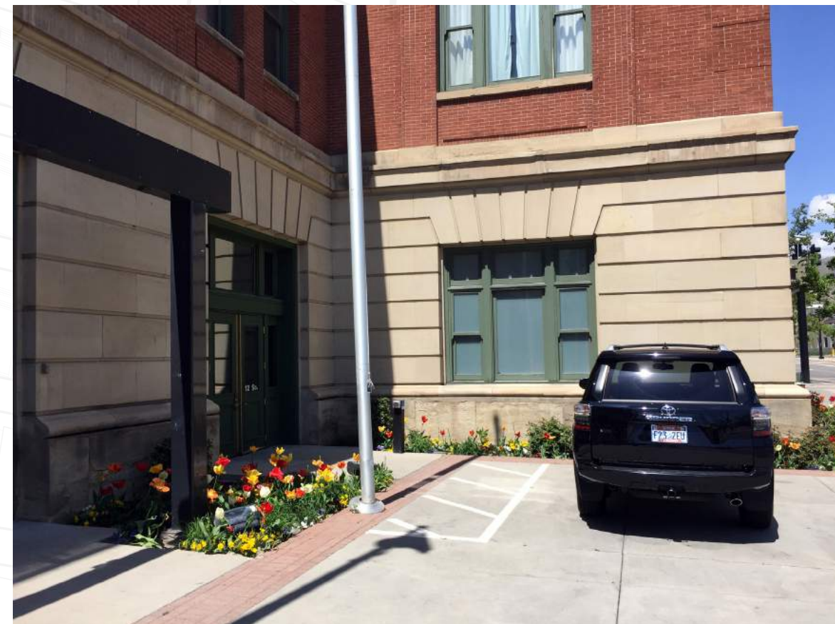
Existing Union Pacific Building base materials and articulation.
