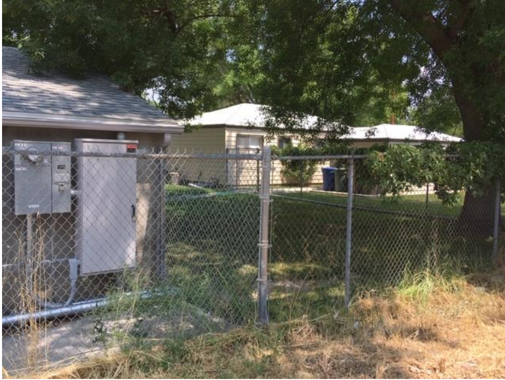
View of the existing antenna electrical equipment towards the rear of the private property looking northeast from the 9-Line Trail
