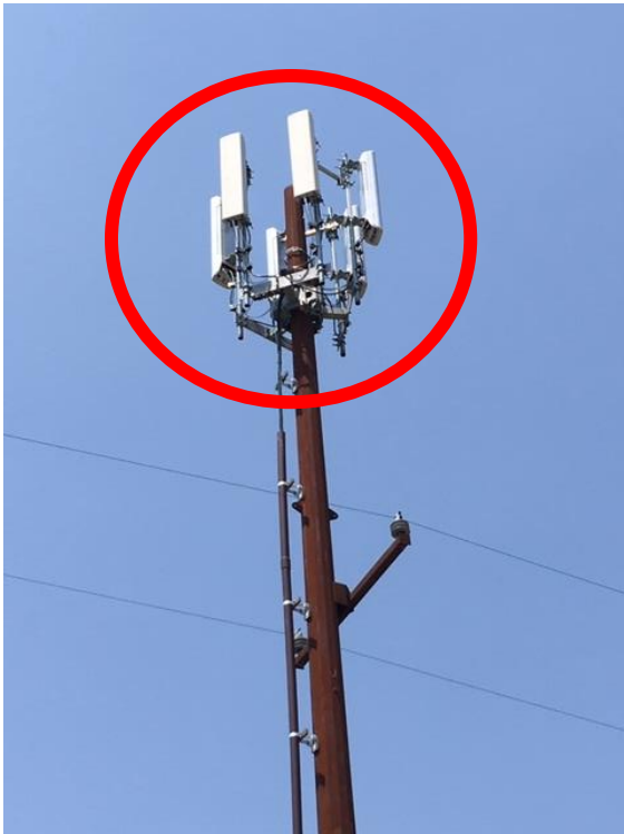
Views of existing antenna array that measures 80” in diameter – to be reduced to 39”
