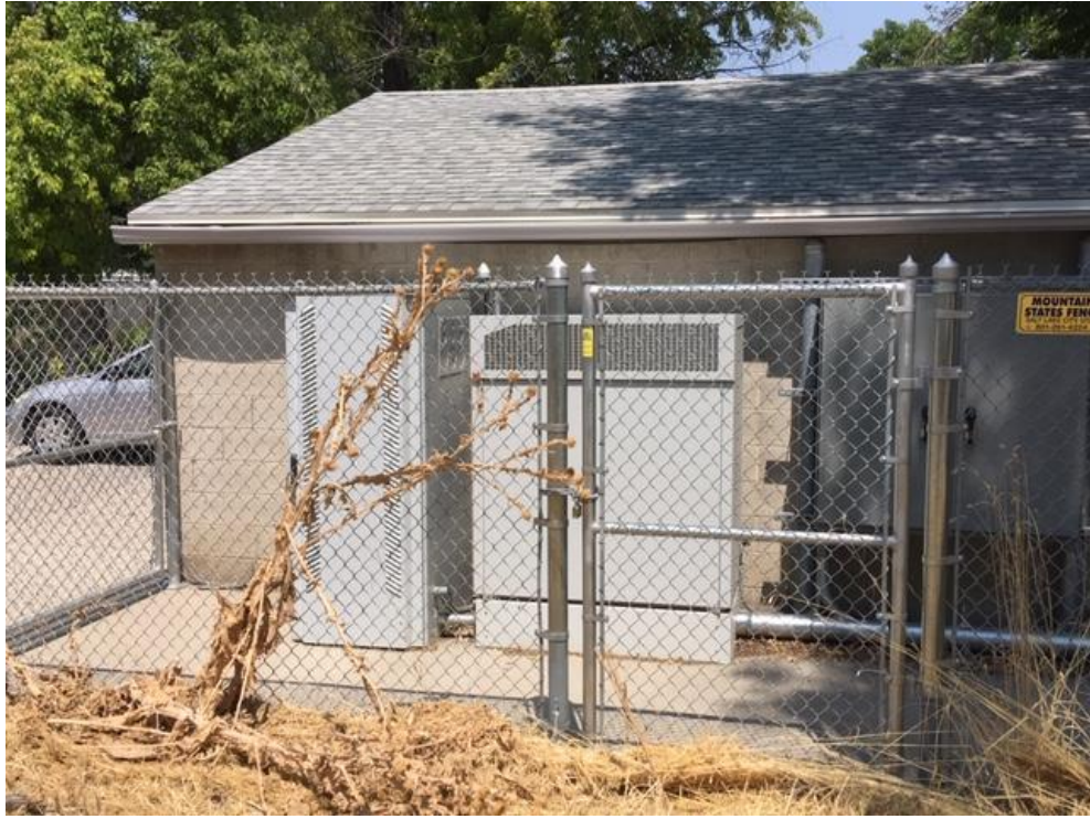
Alternative view of the existing antenna electrical equipment towards the rear of the private property looking northwest from the 9-Line Trail
