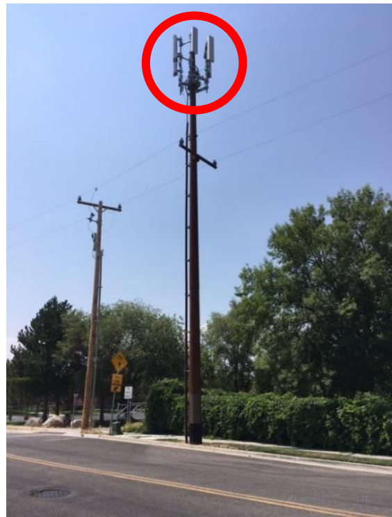
Views of existing antenna array that measures 80” in diameter – to be reduced to 39”
