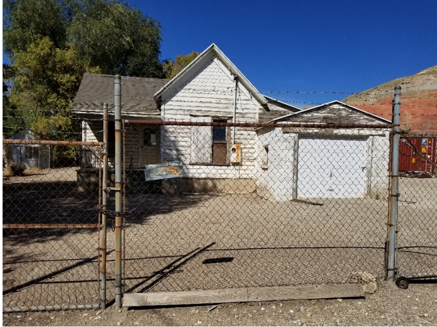
Primary house on the subject property – View looking north
