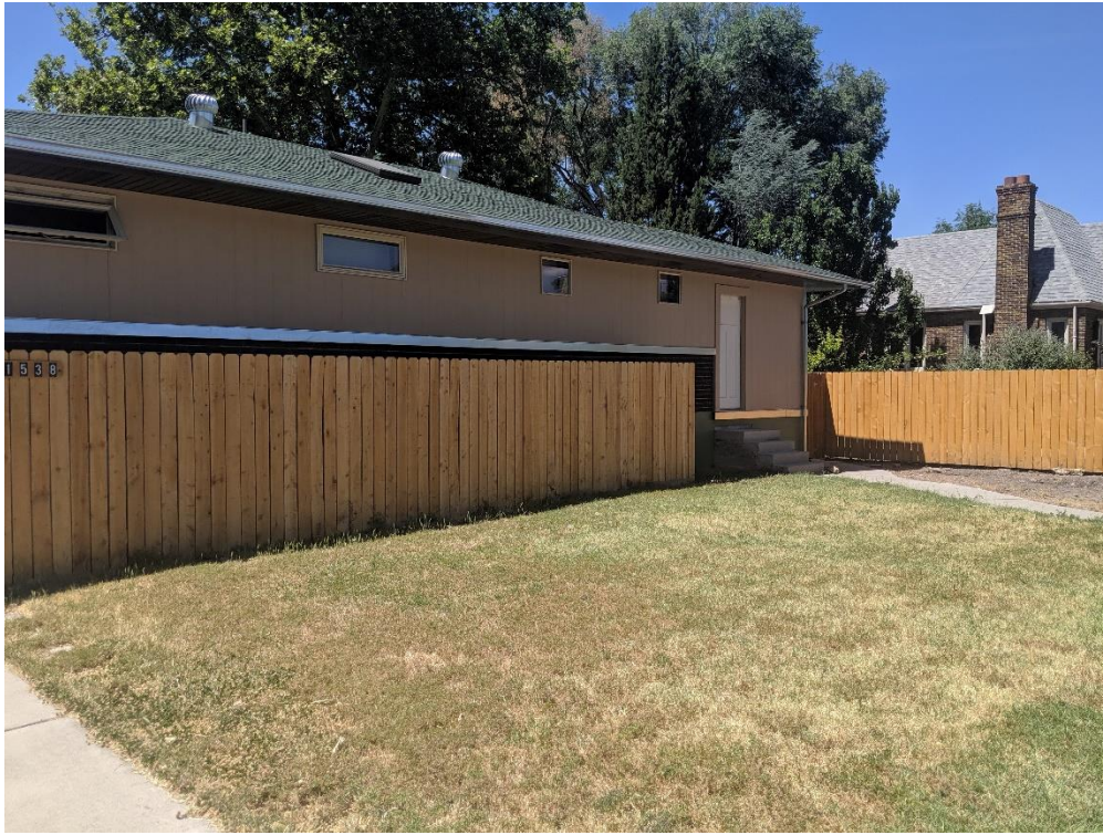
Looking northwest facing the property
